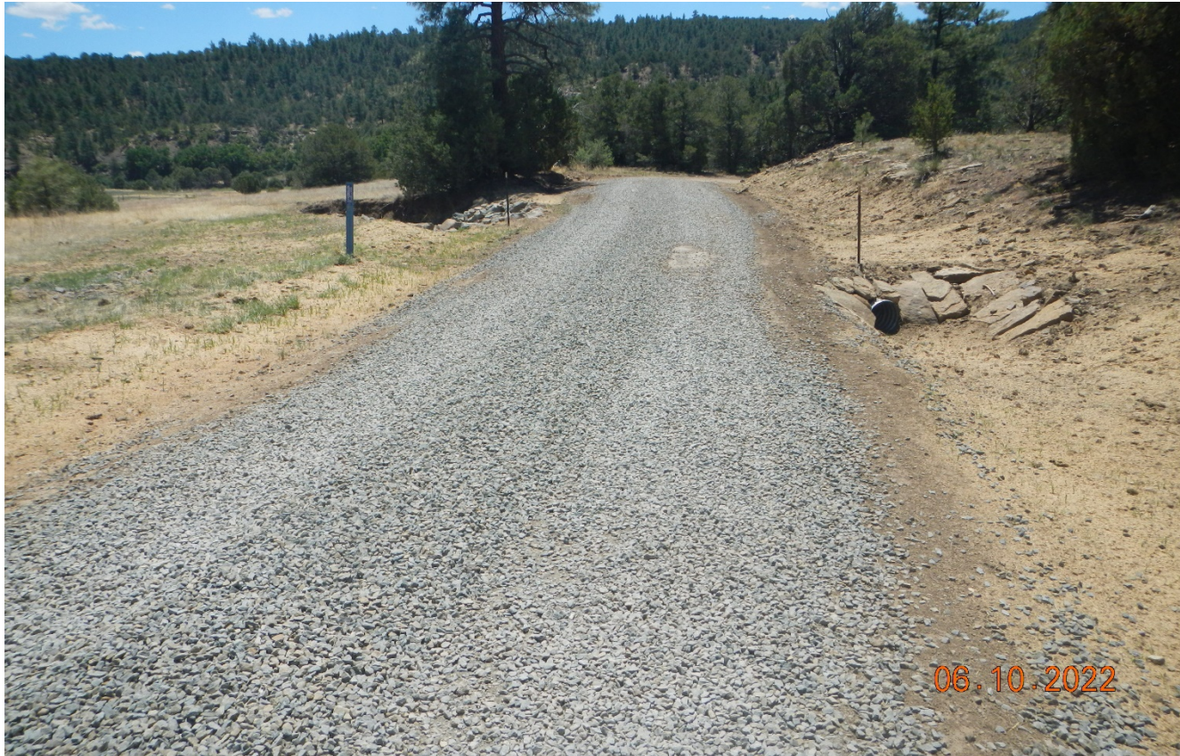
Photo 1. Facing southwest along the main road near the electric gate. The road and culvert has been repaired. Lat/Long:37.08136,-104.62910
