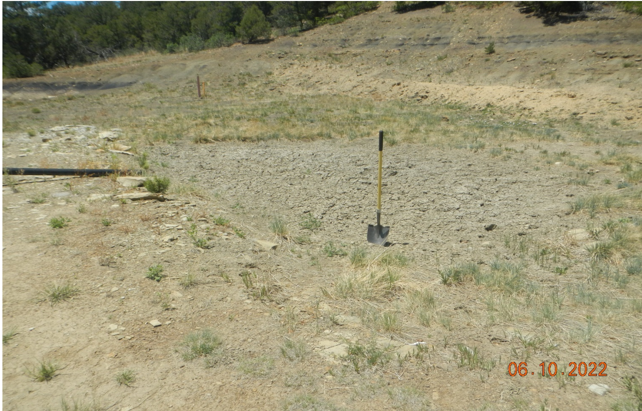
Photo 5. Facing toward the pit.. The pit is shallow; less than 2 ft. deep and needs to be constructed to allow 2 ft. freeboard. Previous corrective action was not completed.
