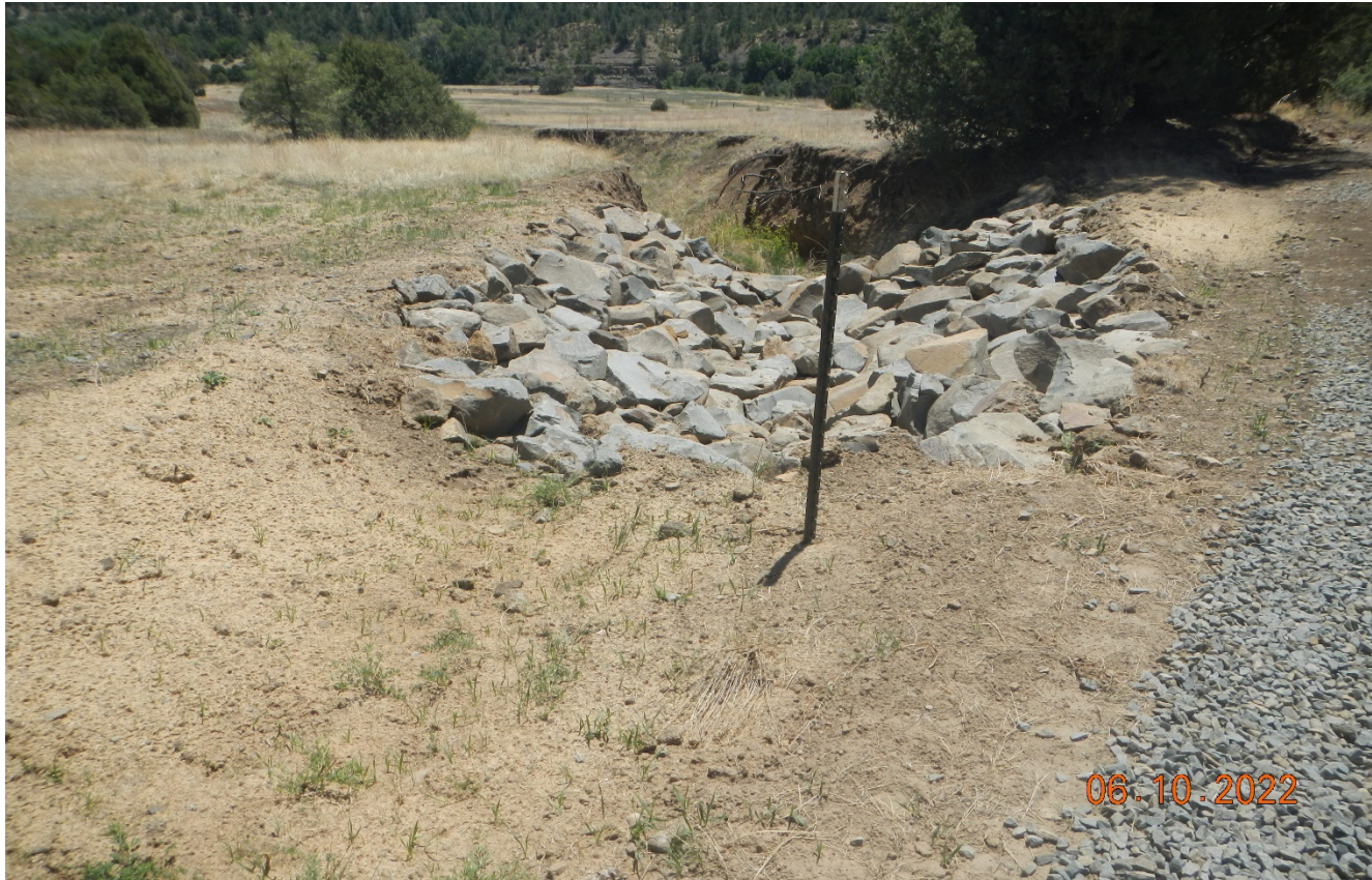
Photo 2. The erosion at the culvert outlet has been repaired with rock rip/rap outlet protection. Areas of disturbance were seeded and hydromulched.
