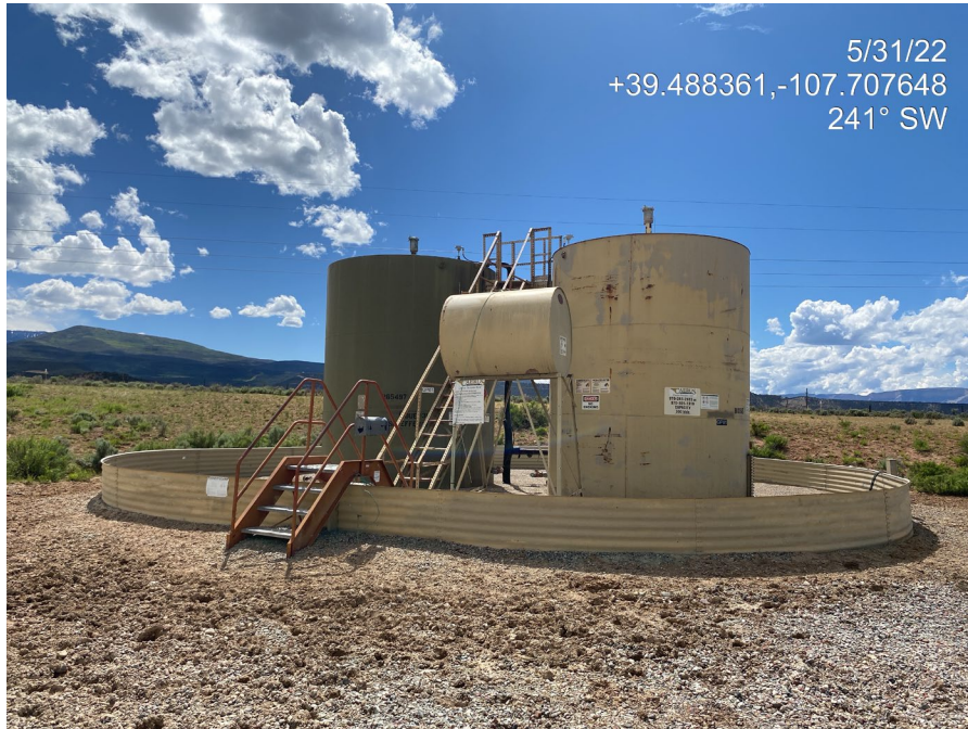
Photo 1. Photo taken from the tank battery at the south of the Location shows a lack of proper signage.
