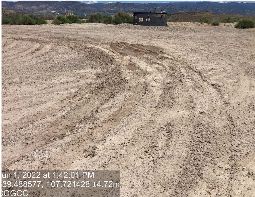
Lack of stabilization/ compaction
