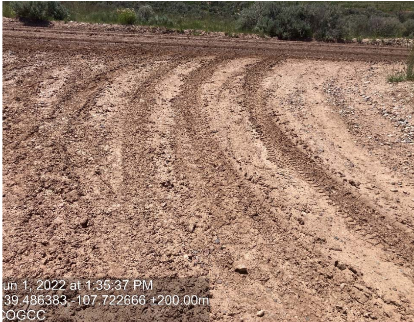
Lack of stabilization/ compaction
