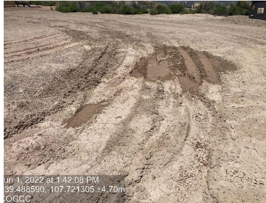
Lack of stabilization/ compaction
