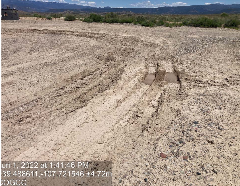
Lack of stabilization/ compaction
