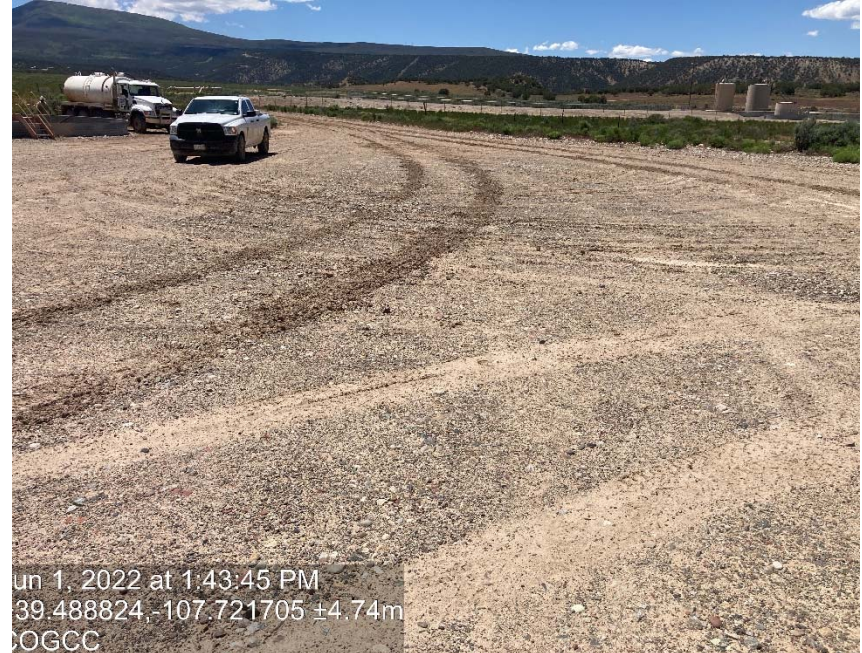
Lack of stabilization/ compaction
