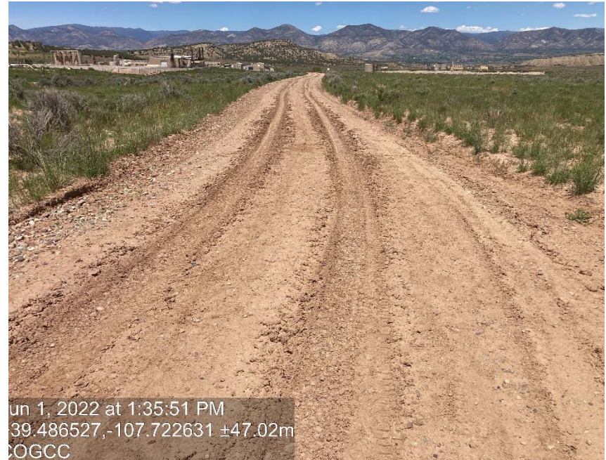
Lack of stabilization/ compaction
