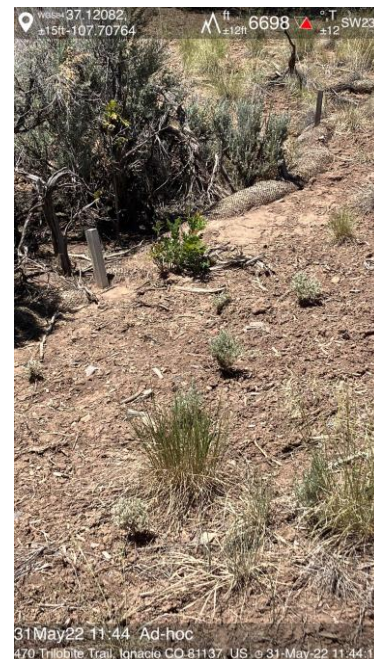
IMG 04 Upslope of waddles filled with sediment
