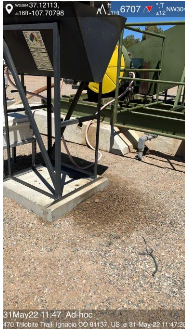
IMG 09 Lube oil has impacted material
