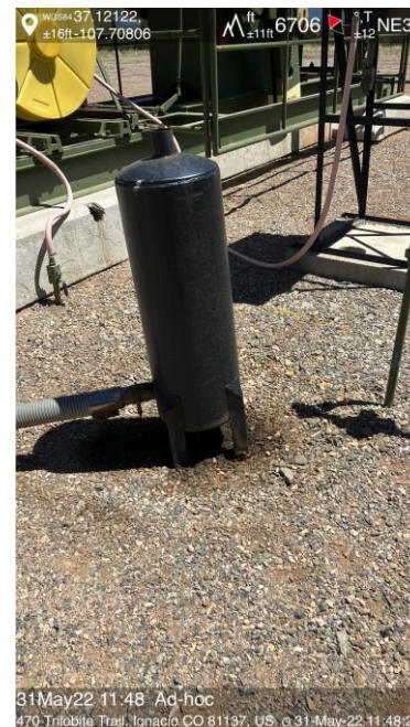
IMG 12 Exhaust muffler has impacted material
