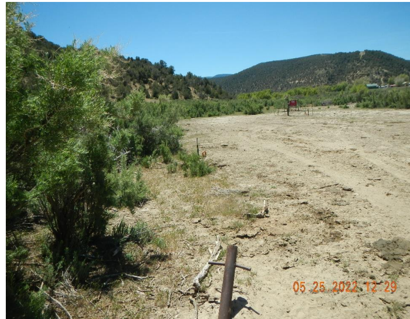
Unmarked anchor and Markers that aren't 4' and brightly colored.
