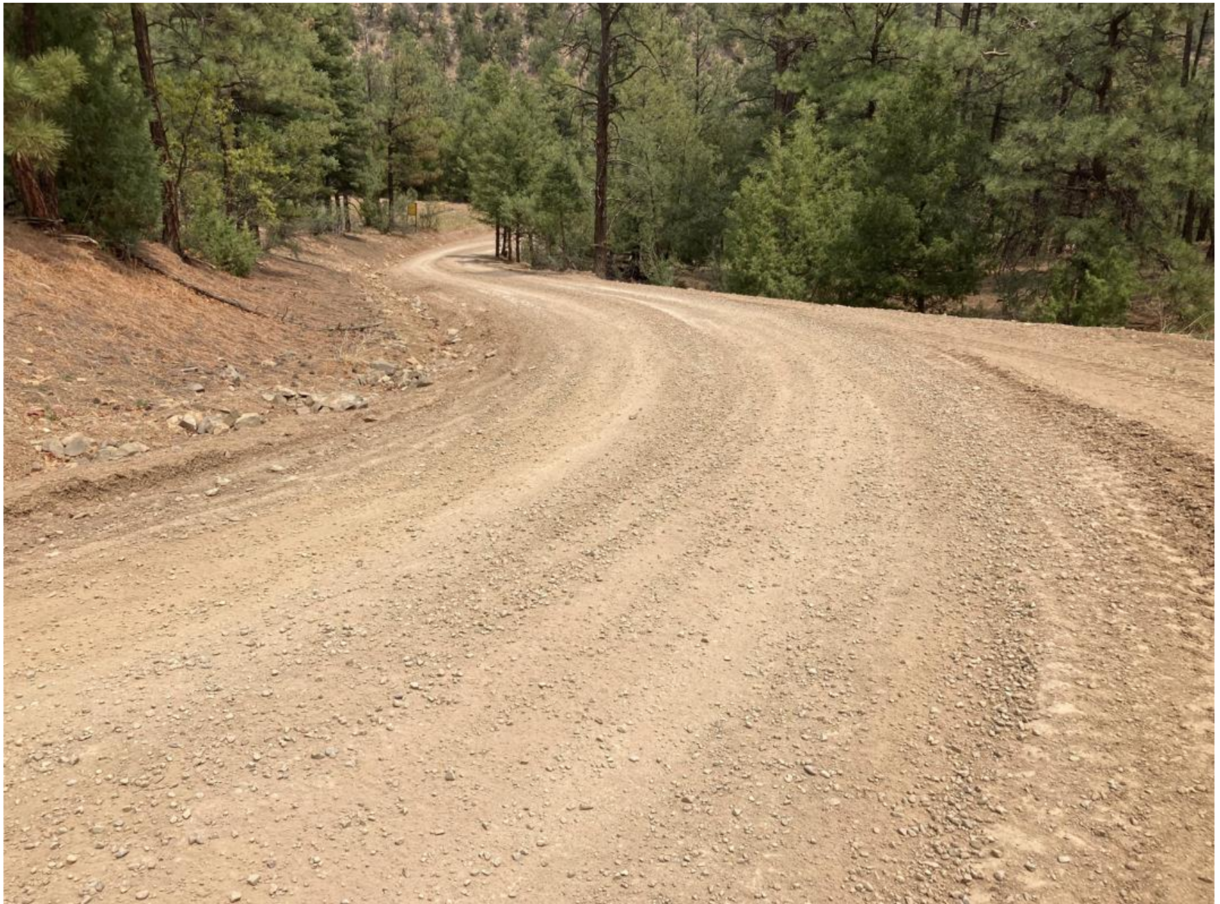
PHOTO 4: THE TIRE RUTS ON THE SIDE OF JEEP TRAIL LEASE ROAD WERE REGRADED TO CREATE SHEET FLOW. GRAVEL WAS INSTALLED IN THIS AREA FOR ROADWAY SOIL STABILIZATION. ROCK CHECK DAMS HAVE BEEN INSTALLED IN THE DIVERSION DITCH ALONGSIDE THE ROAD.
