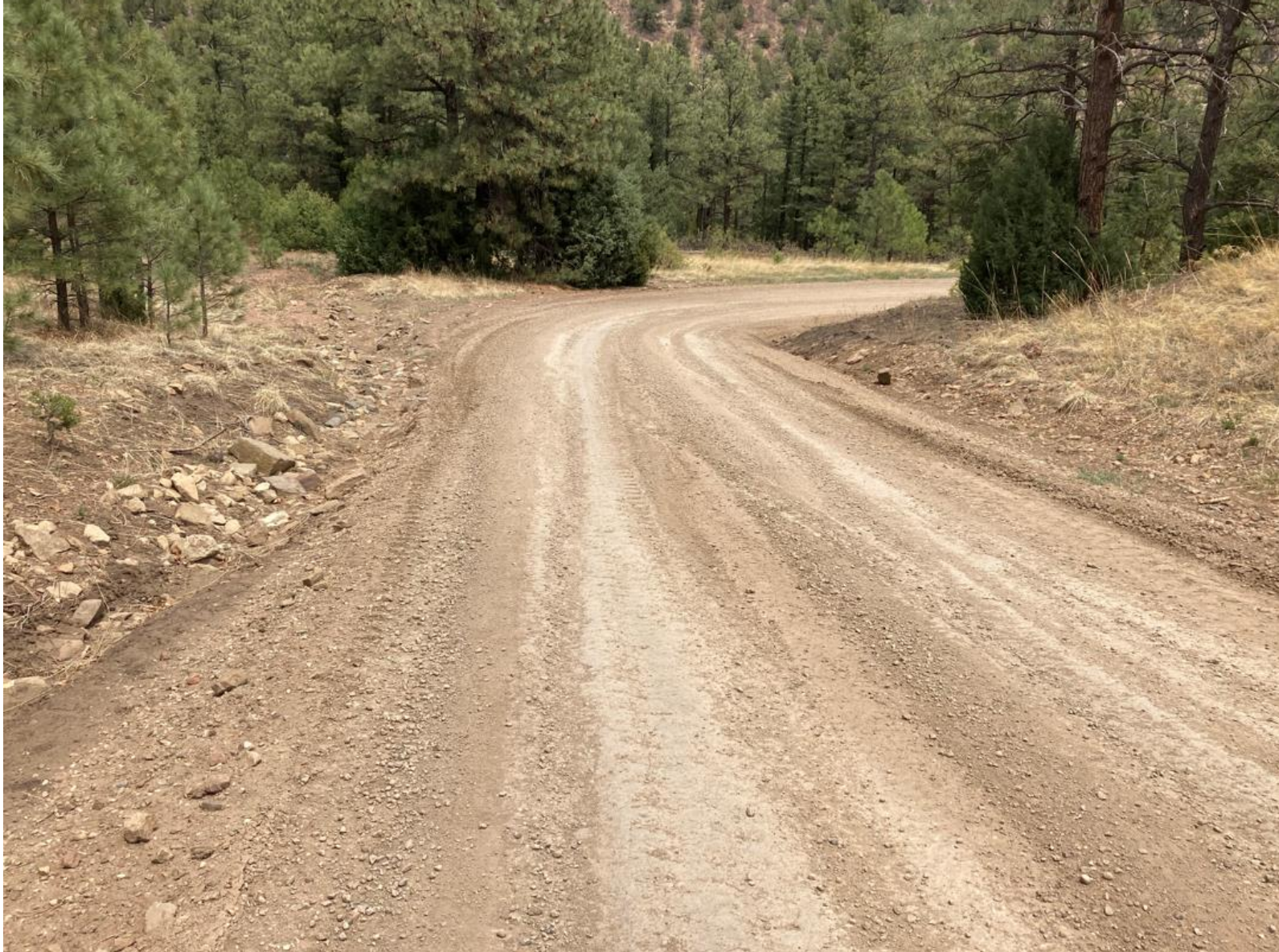
PHOTO 1: THE JEEP TRAIL LEASE ROAD WAS SURFACED CROWNED TO CREATE SHEET FLOW. ADDITIONAL GRAVEL WAS INSTALLED FOR ROADWAY SOIL STABILIZATION.
