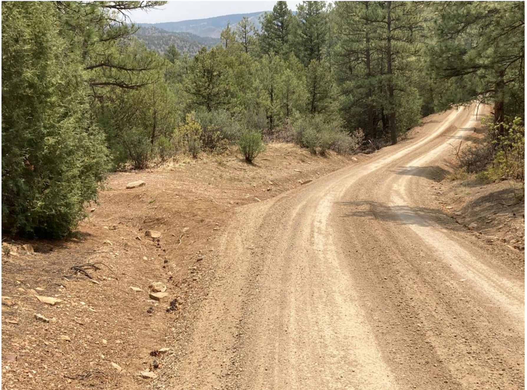
PHOTO 6: THE JEEP TRAIL ROAD SURFACE WAS REGRADED TO ELIMINATE THE TIRE RUTS. ADDITIONAL GRAVEL WAS INSTALLED FOR ROADWAY SOIL STABILIZATION. DIVERSION DITCHES AND TURNOUTS HAVE BEEN REDEFINED TO PROPERLY DIVERT STORMWATER RUNOFF.
