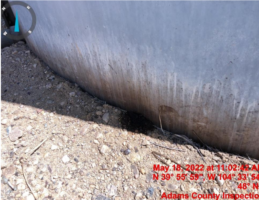
Photo#5 Potential pinhole in production tank. Stained Soil
