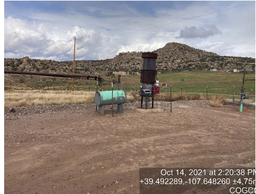
Stored equipment (ECD is disconnected from tanks and gas) From previous inspection (10/14/2021)
