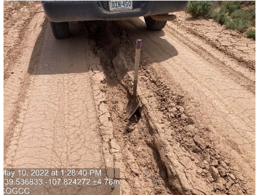
Lack of stabilization/compaction/ degradation
