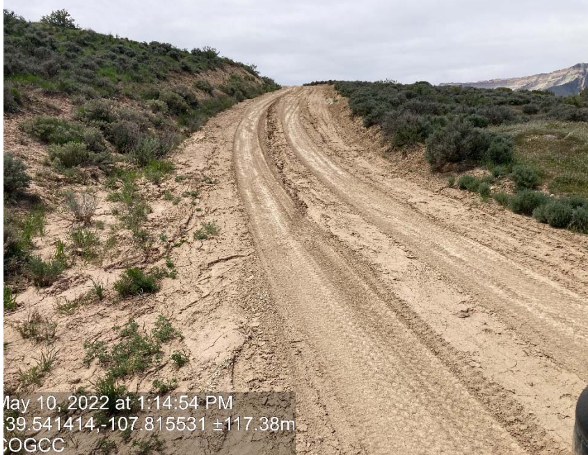
Lack of stabilization/compaction/ degradation
