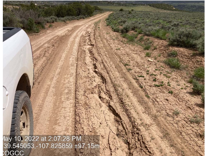
Lack of stabilization/compaction/ degradation
