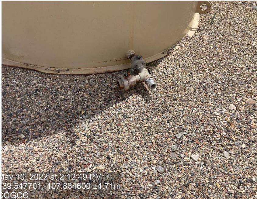
Valve missing caps/plugs
