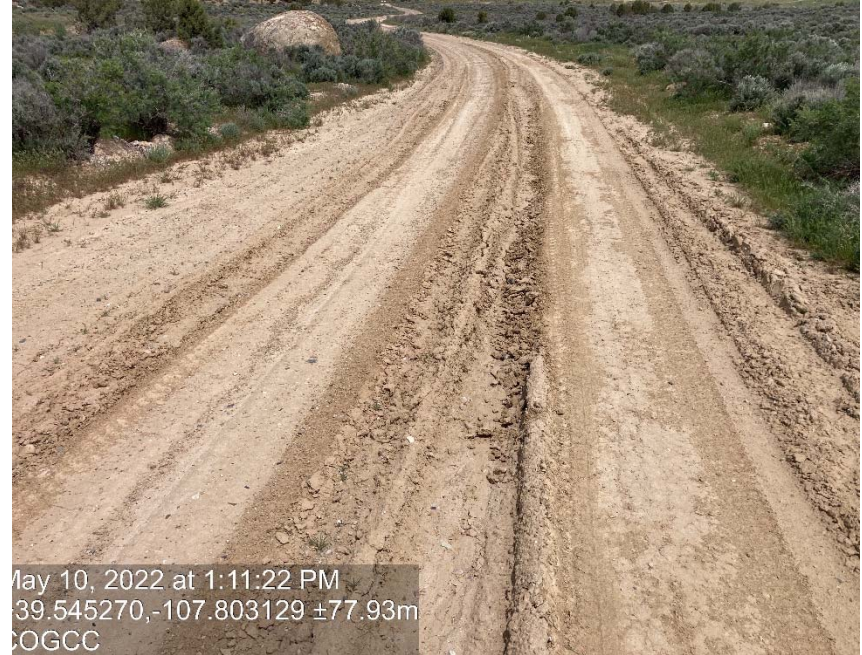
Lack of stabilization/compaction/ degradation
