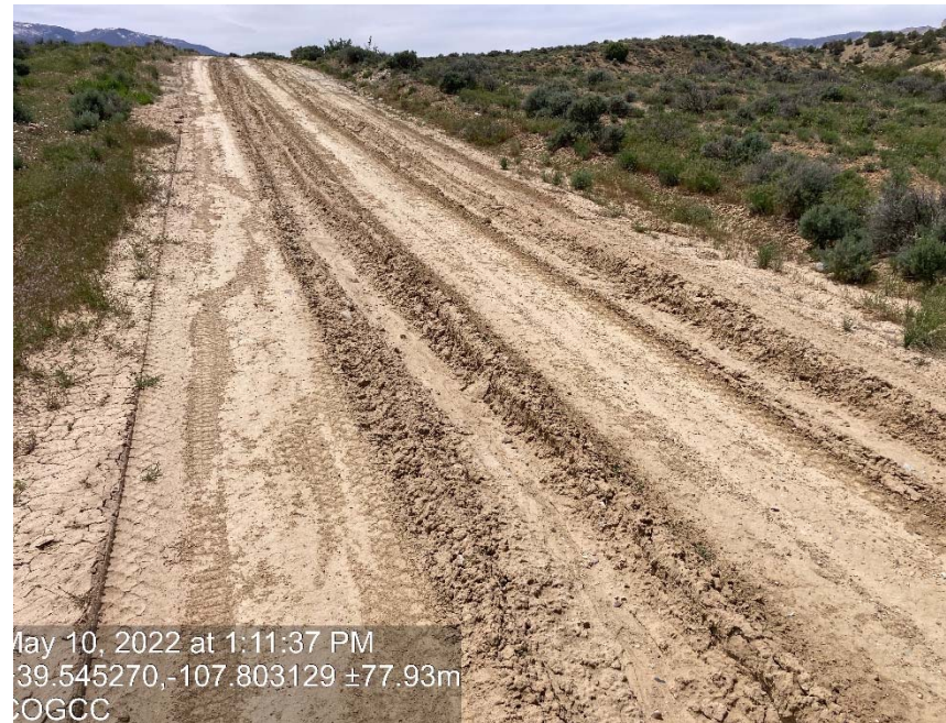
Lack of stabilization/compaction/ degradation
