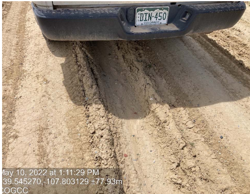
Lack of stabilization/compaction/ degradation
