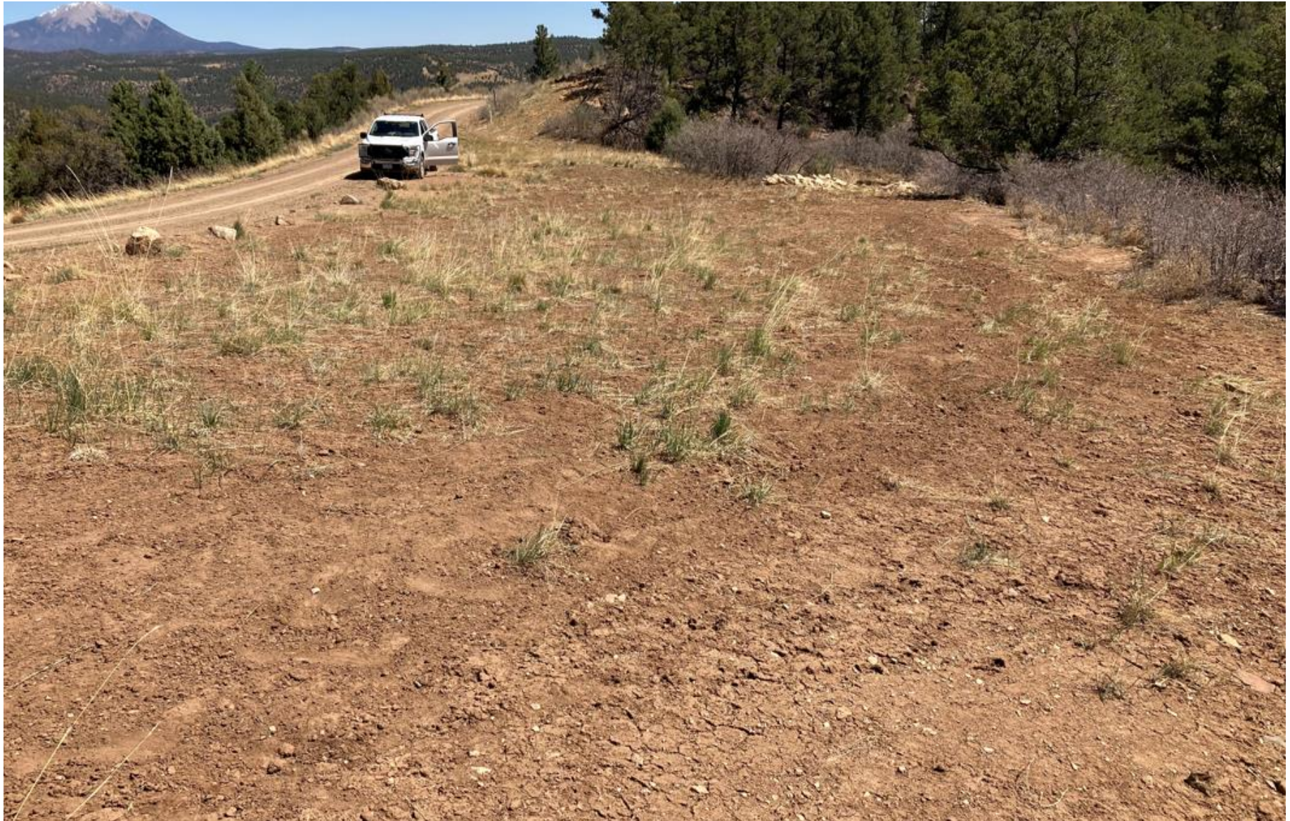
PHOTO 2: THE TIRE RUTS AND RILLING HAVE BEEN HAND RAKED.
