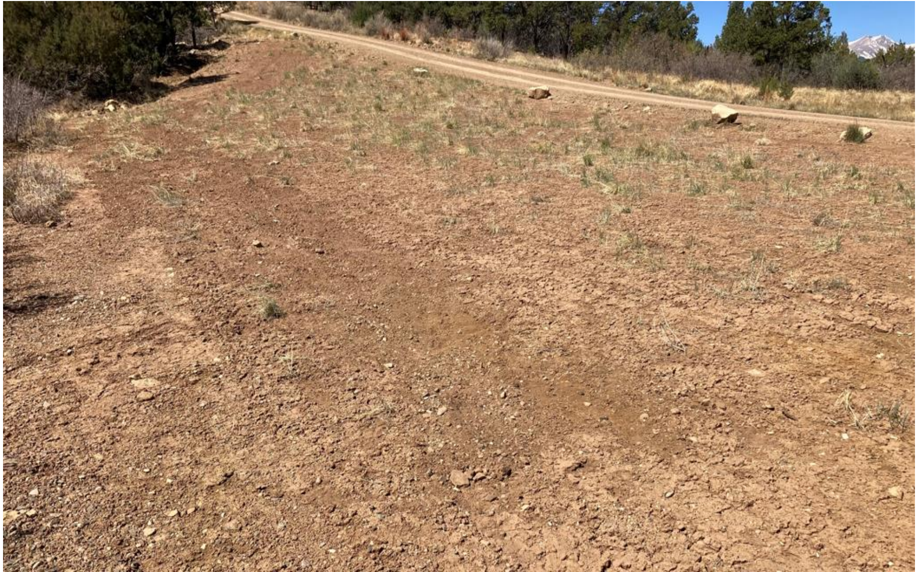
PHOTO 1: THE TIRE RUTS AND RILLING HAVE BEEN HAND RAKED.
