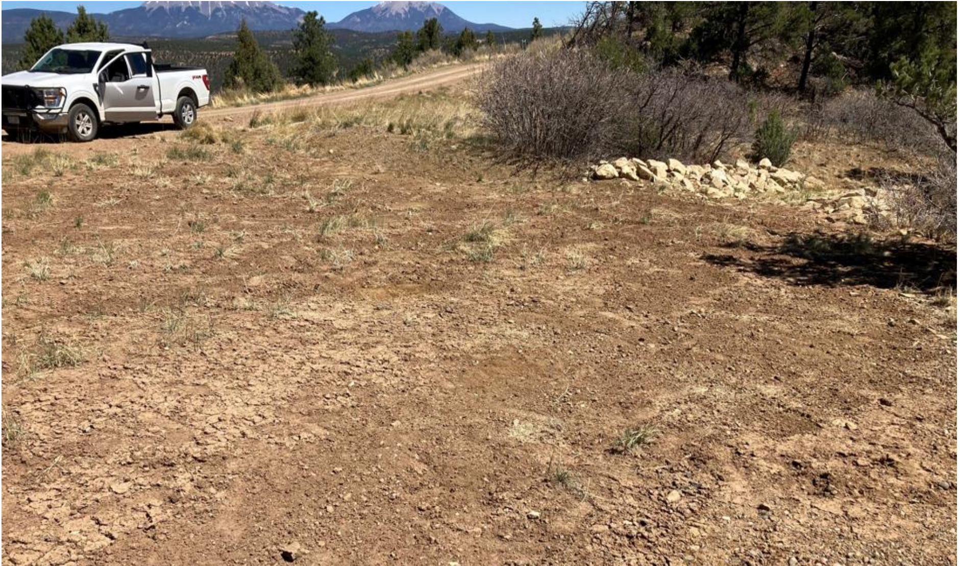
PHOTO 3: THE TIRE RUTS AND RILLING HAVE BEEN HAND RAKED. THE DIVERSION DITCH HAS ALSO BEEN CLEANED OF SEDIMENT AND REDIFIED TO DIVERT STORMWATER TO THE ROCK SPILLWAY.
