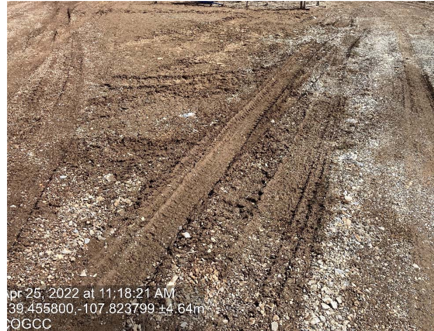
Lack of stabilization/compaction
