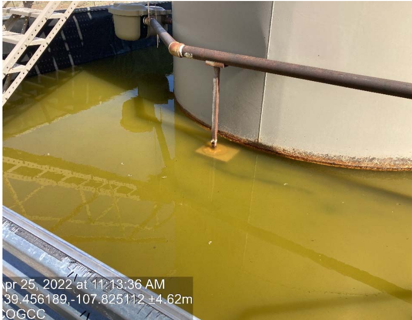
Stained fluid in containment
