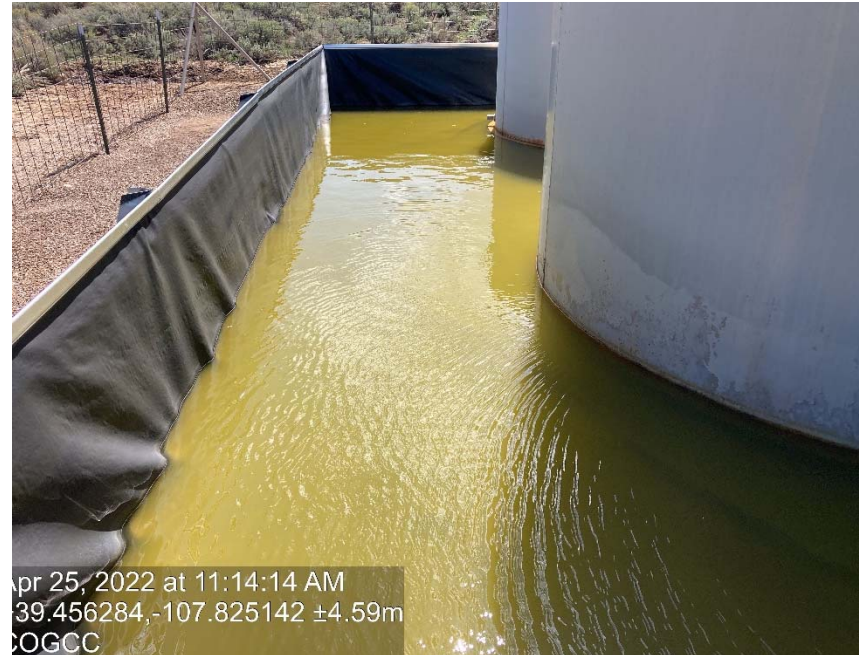
Stained fluid in containment
