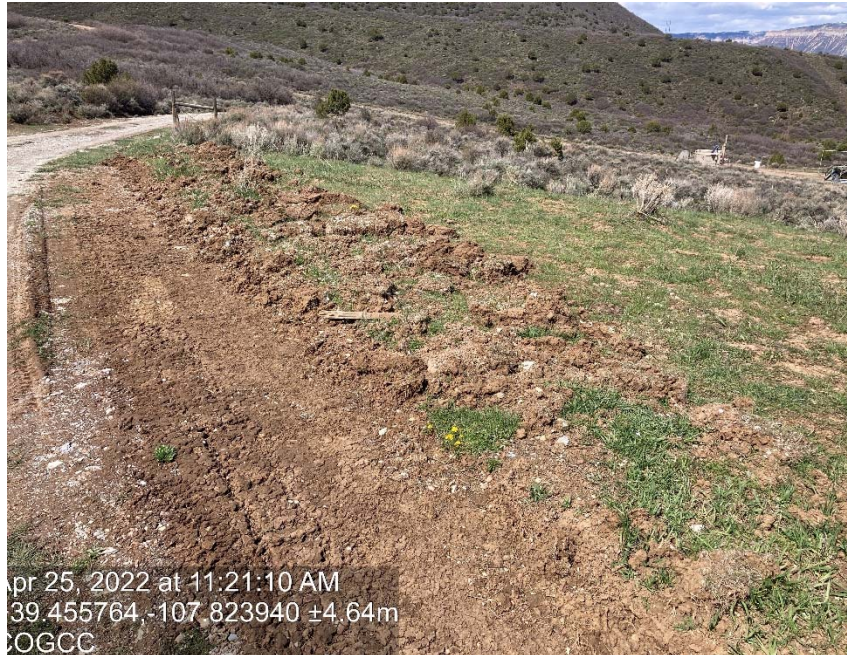
Sediment pushed off of access/location
