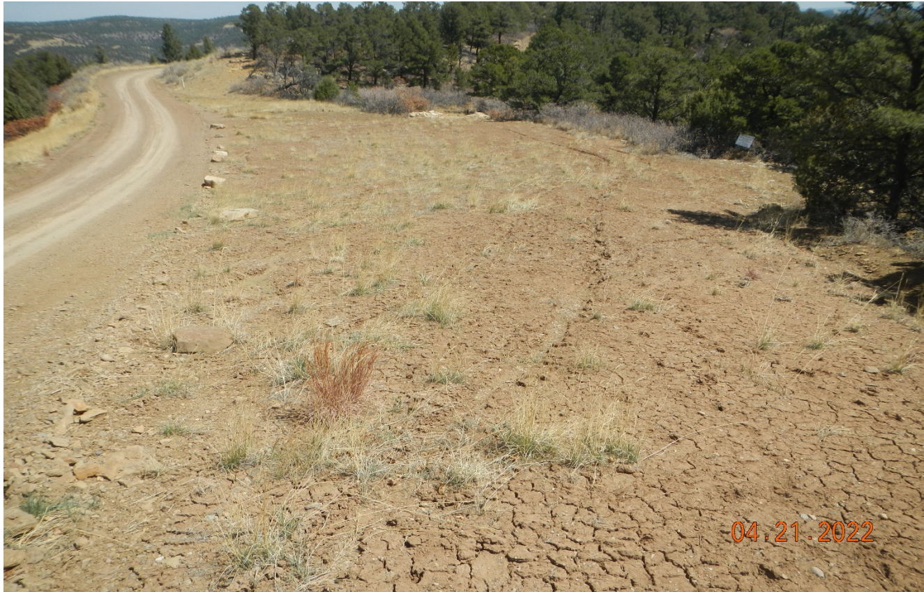
Photo 1. Facing northeast toward the abandoned location. Additional seeding needs to be performed in this area.
