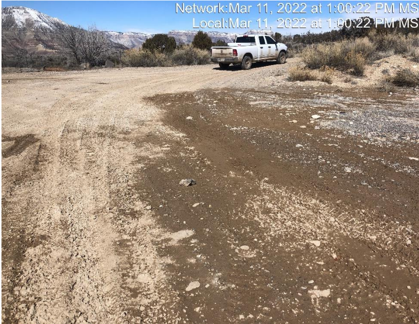
Photo #6155 Insufficient tracking controls at entrance to location.
