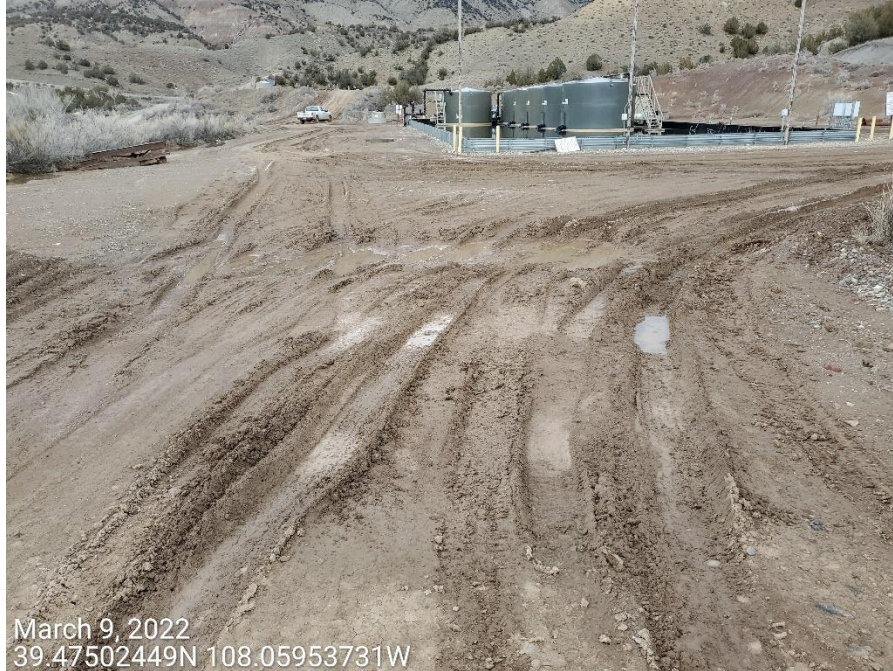
Photo 4: Photo example showing control measures to address stabilization and tracking on the Location are missing or insufficient.
