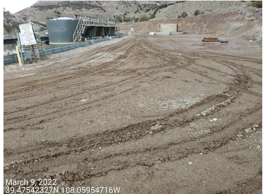
Photo 3: Photos example showing control measures to address stabilization and tracking on the Location are missing or insufficient.
