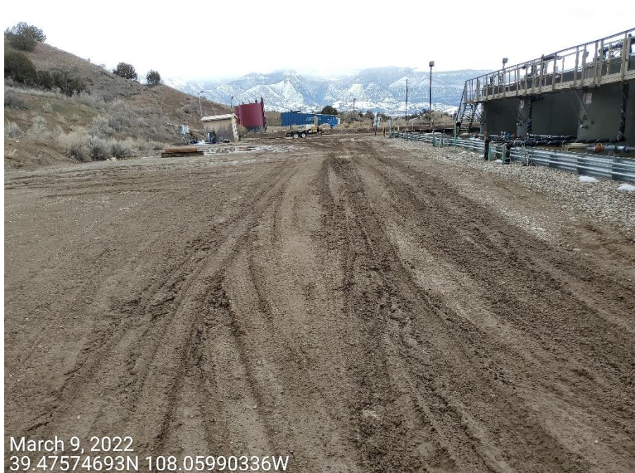
Photo 3: Photos example showing control measures to address stabilization and tracking on the Location are missing or insufficient.
