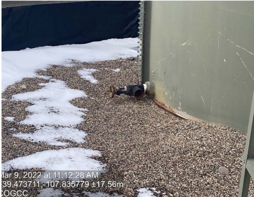
Valve missing cap/plug
