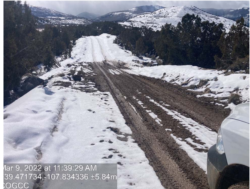
Lack of stabilization/compaction
