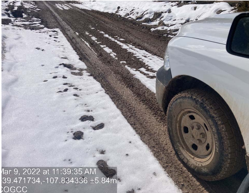
Lack of stabilization/compaction
