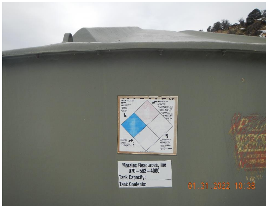
Tank label does not meet required information.
