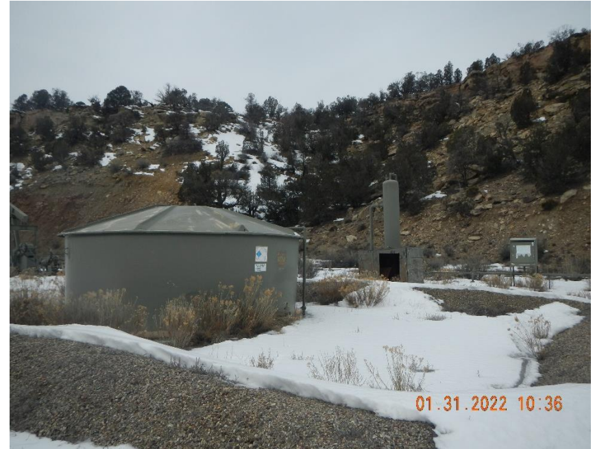
Weeds growing inside of tank berm.
