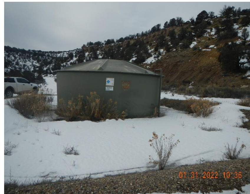
Weeds growing inside of tank berm.
