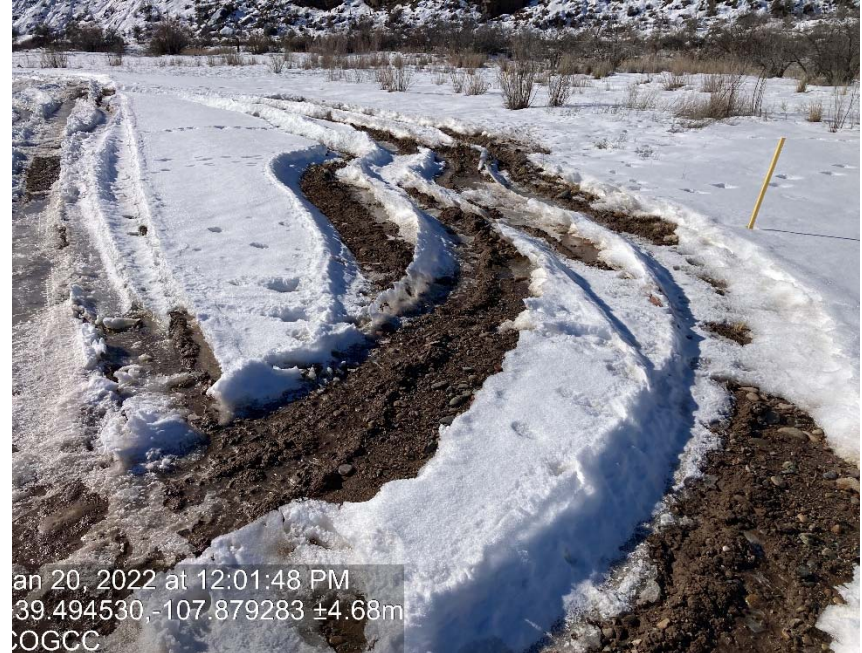
Lack of stabilization/compaction
