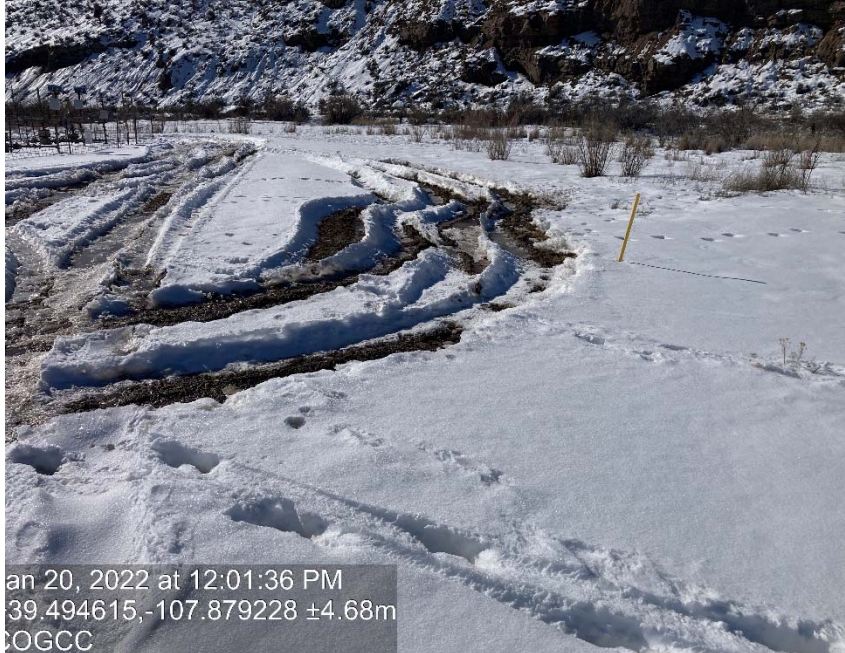
Lack of stabilization/compaction
