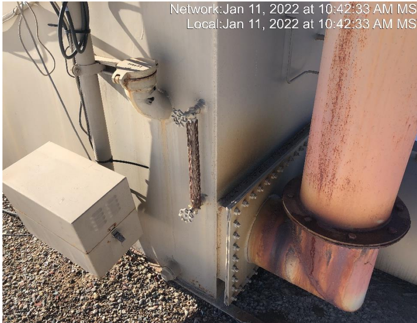
Photo #5642 Sight glass indicates the storage tank is full of an unknown fluid.
