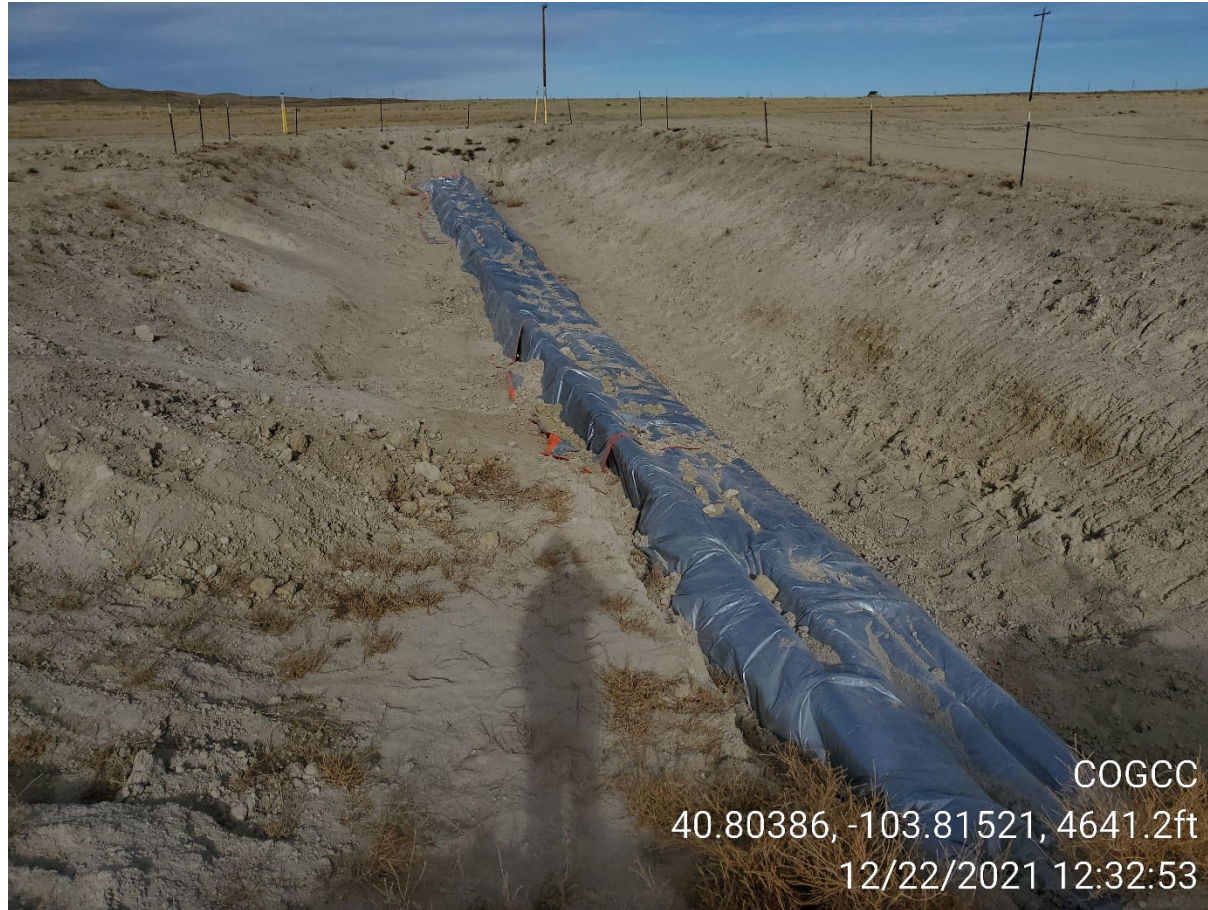
Photo 1 Open excavation at flowline spill just north of Razor 25N location
