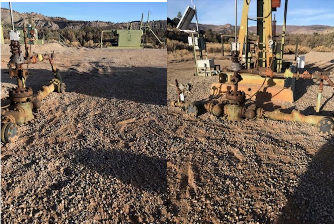
Well head and impacted soil cleaned up and repaired.
