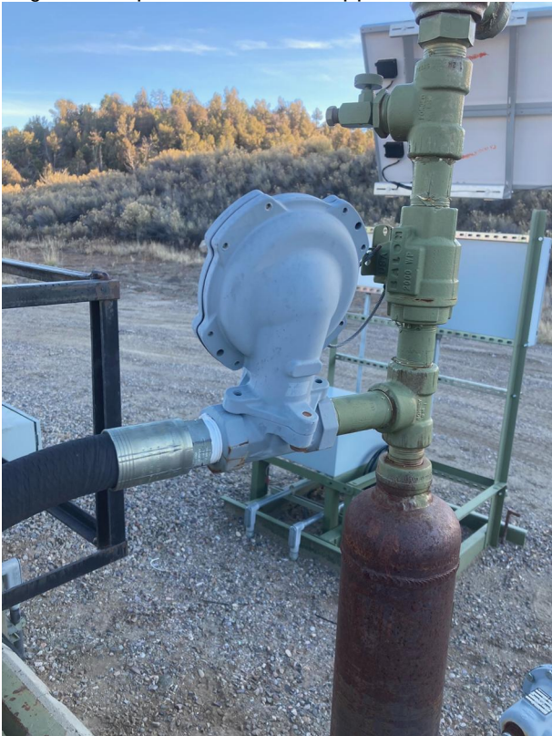
Regulator repaired and leak stopped.
