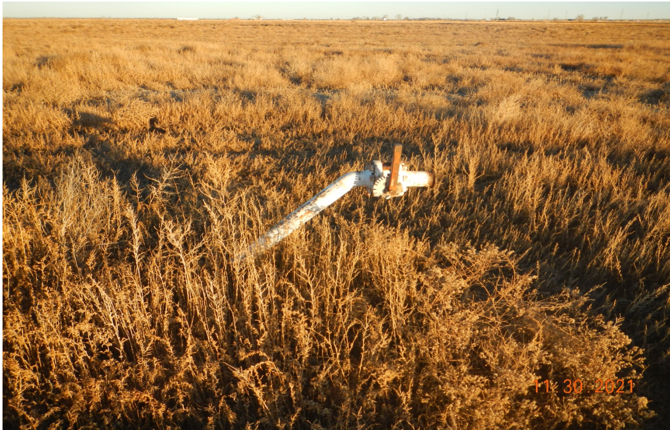
Photo 1. There is abandoned pipe riser that remains at the location which needs to be removed.
