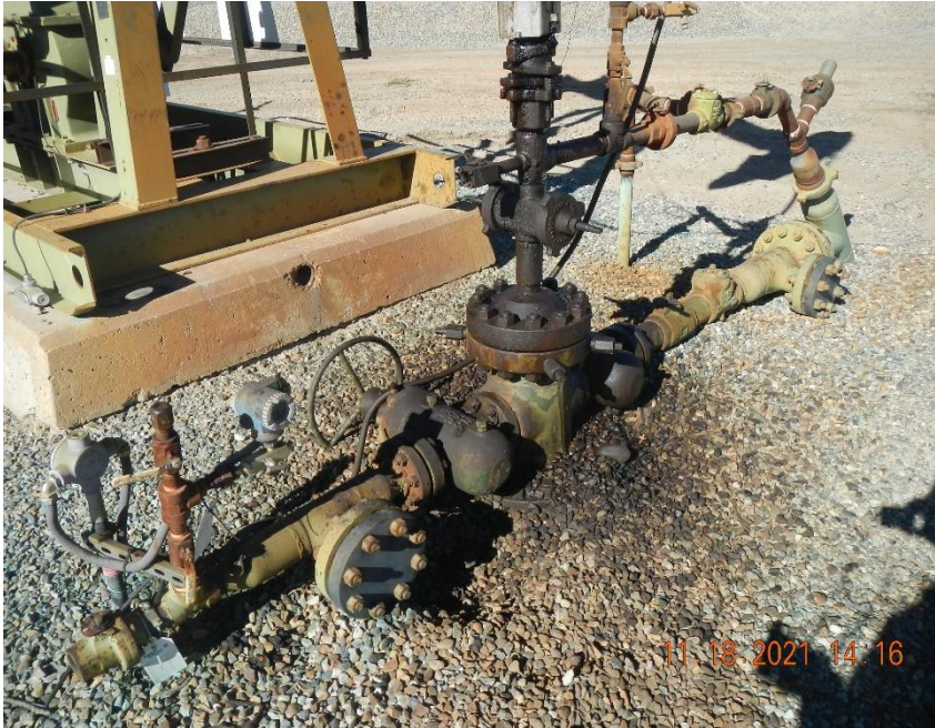
Well head and surrounding area are wet and stained.
