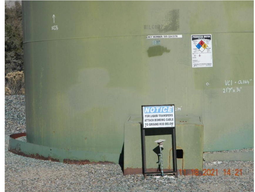
AST signage is not compliant with Rule 605.h.
