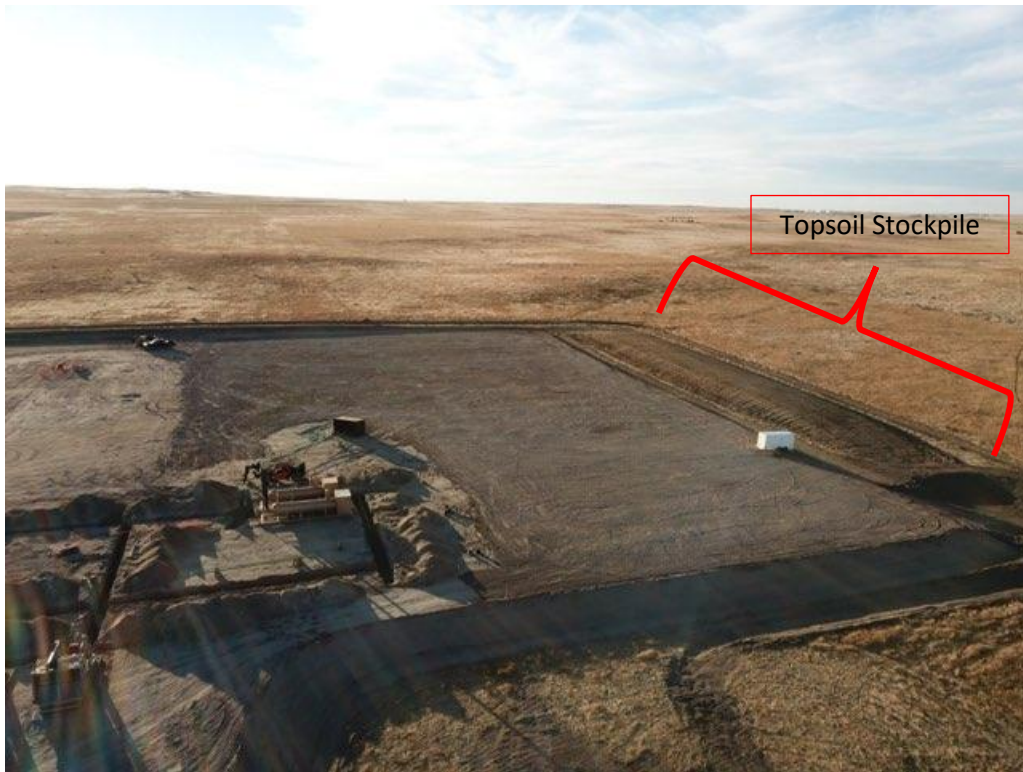
Aerial photo showing topsoil stockpile and completed road base application
