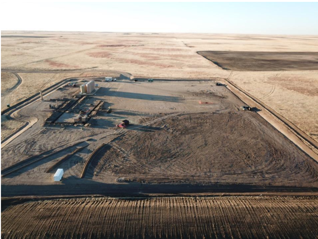
Applying additional road base to uncovered portion of the pad (in-progress)
