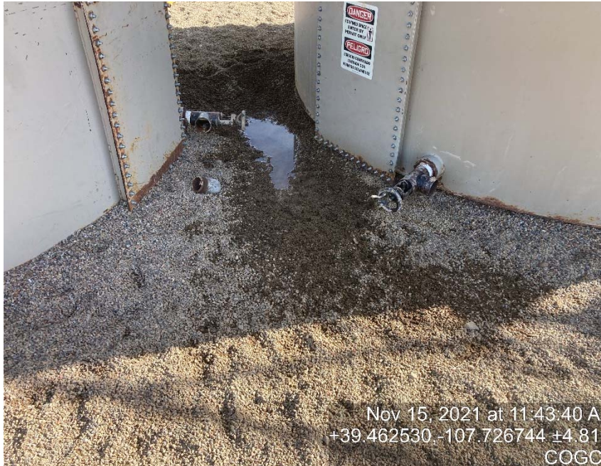
Staining/load out lines
