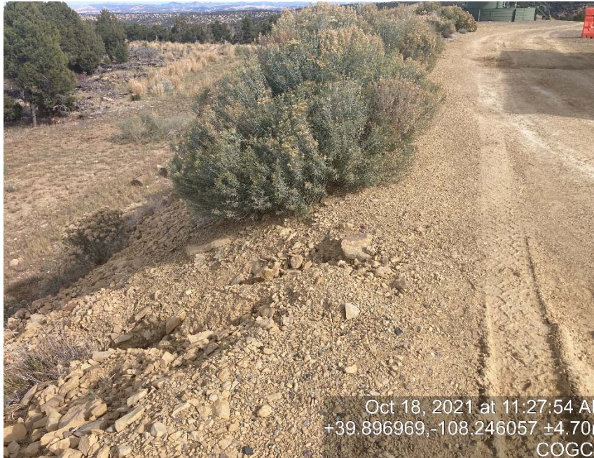
Fill slope erosion
