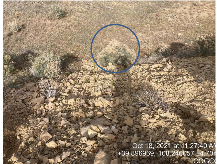
Fill slope erosion/sediment migration
