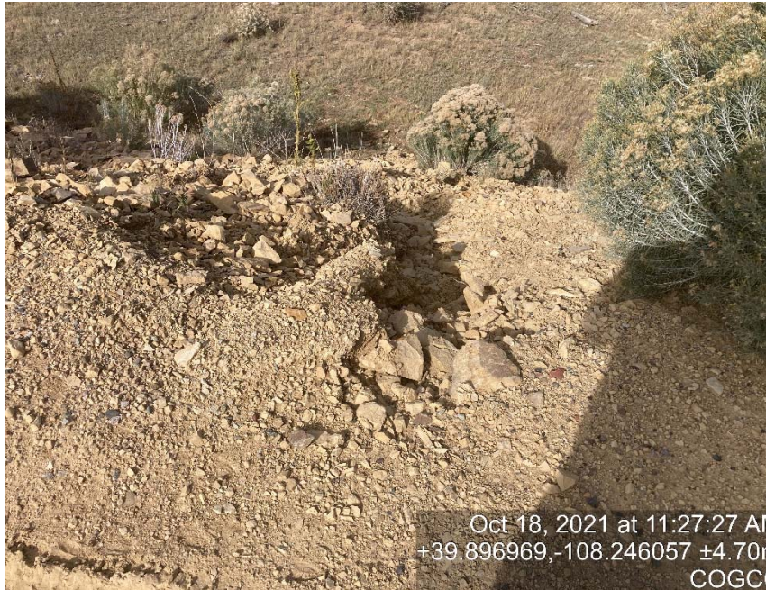
Fill slope erosion
