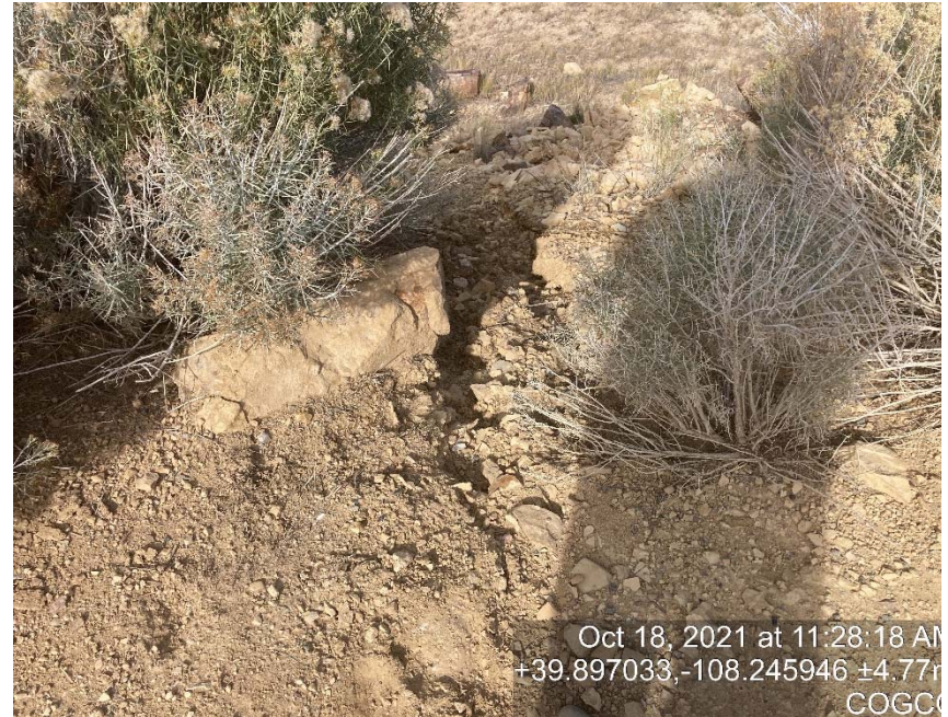
Fill slope erosion
