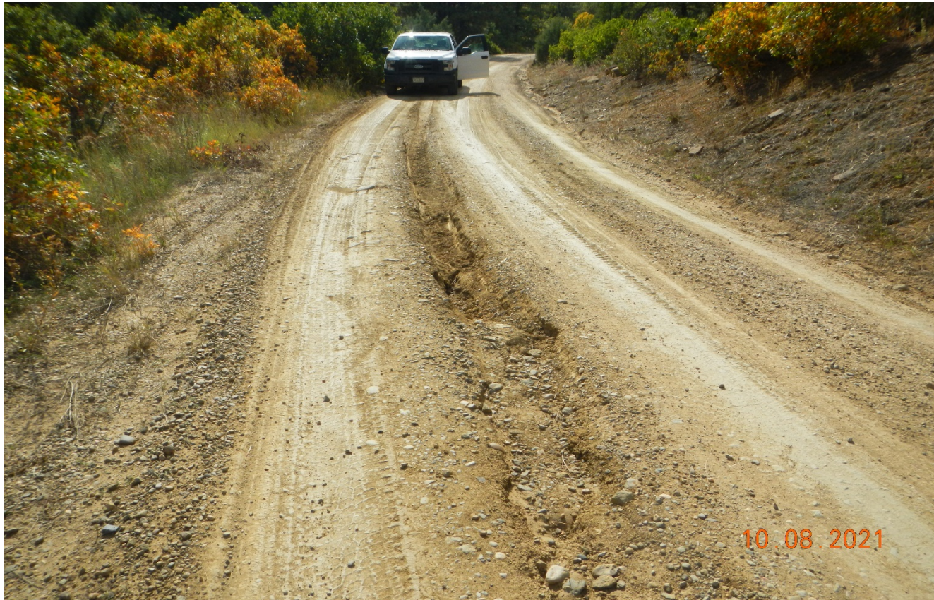
Photo 3. Further along the road is erosion channeling along the center of the road. Areas of erosion and vehicle rutting need to be repaired and stabilized.
