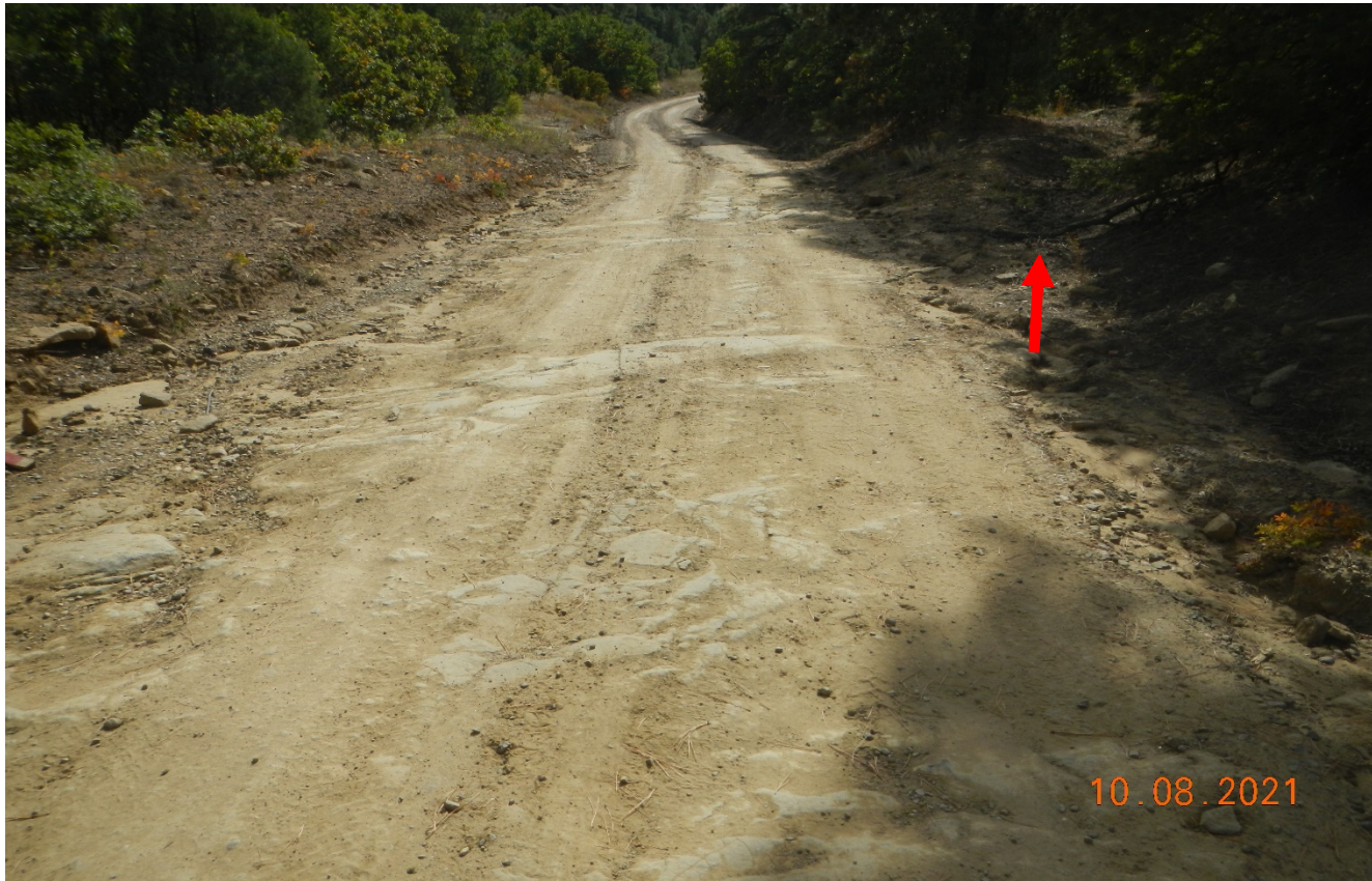
Photo 5. Similarly to previous photo, stormwater is not properly diverted at red arrow. This area of the road is not stabilized.
