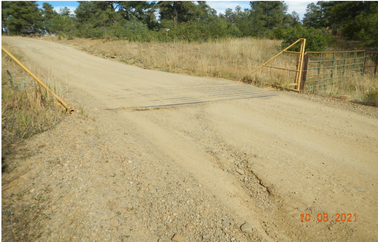
Photo 6. There is a cattleguard that is filled in with sediment at Lat/Long: 37.24379,-104.68923.
