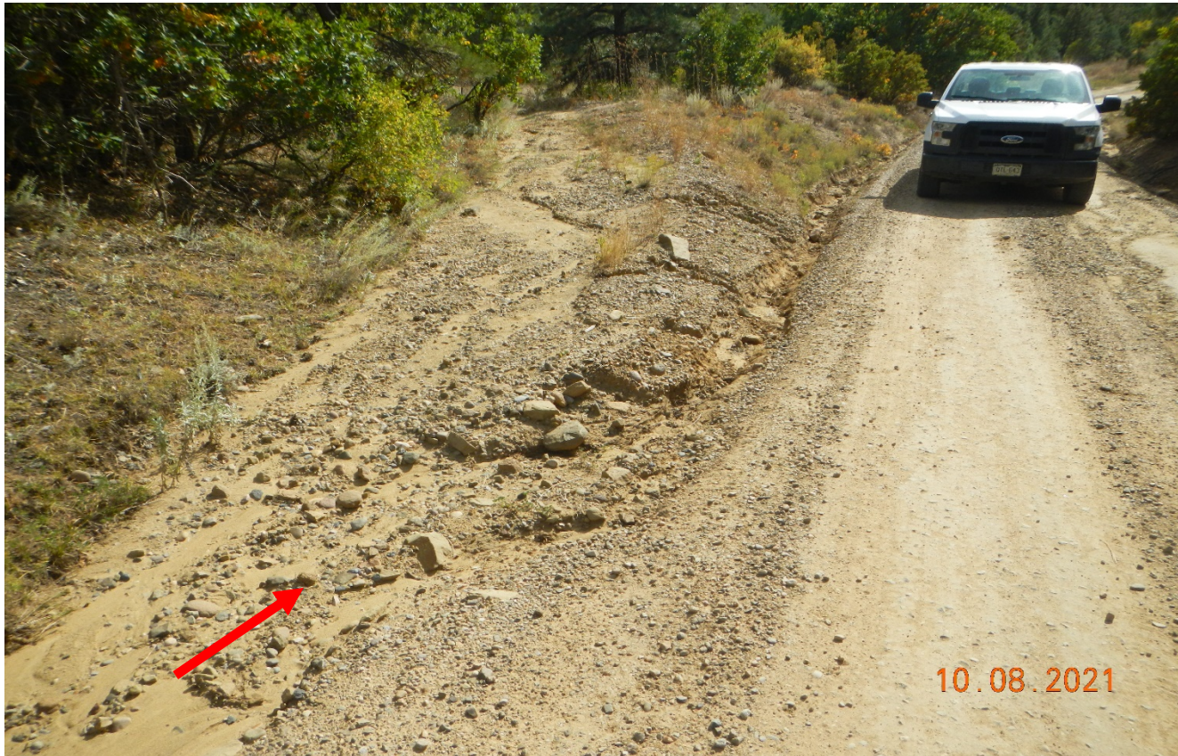
Photo 4. This area of stormwater diversion has filled in with sediment causing erosion to occur down the road side shown at red arrow. The stormwater diversion needs to be repaired with proper BMP installation such as a sediment trap.
