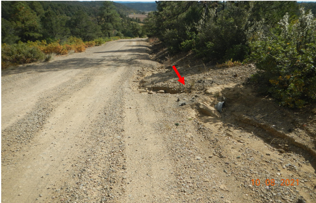
Photo 2. Further along the road toward the location are areas of erosion that need to be repaired. Stormwater is flowing past the culvert shown at red arrow. Lat/Long:37.23760,-104.69906.
