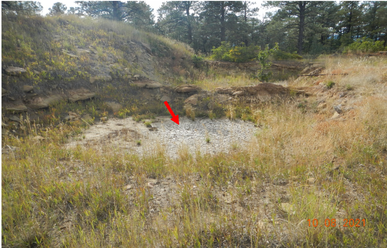
Photo 9. Facing toward the pit. The portion of the pit shown at red arrow appears to be drilling mud in the pit that needs to be cleaned up.
