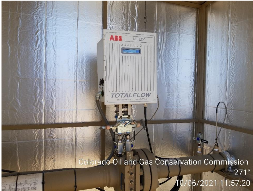
Photo 7 – Calibration Card is Missing
