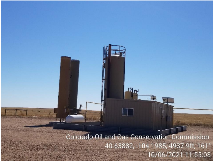
Photo 3 – Heater Treater and ECDs
