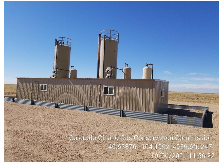
Photo 6 – West Heater Treaters
