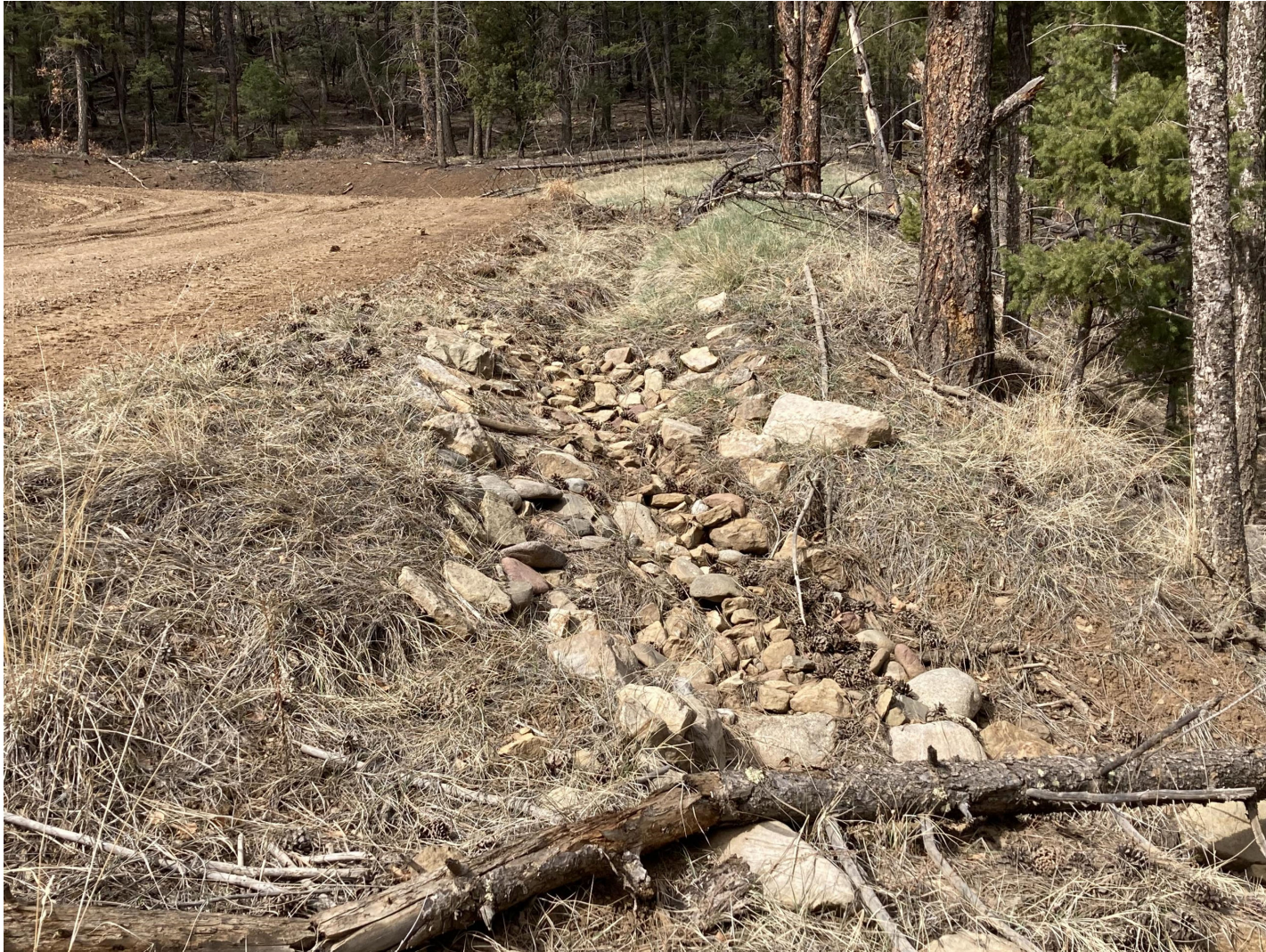
PHOTO 2: THE ROAD SURFACE WAS CROWNED TO CREATE SHEET FLOW AND ELIMINATE THE TIRE RUTS. STORMWATER RUN OFF FROM THE ACCESS ROAD IS DIRECTED TO THE EXISTING ARMORED CALL OUT WHICH IS UPGRADIENT OF A CULVERT ON THE MAIN ROAD.
