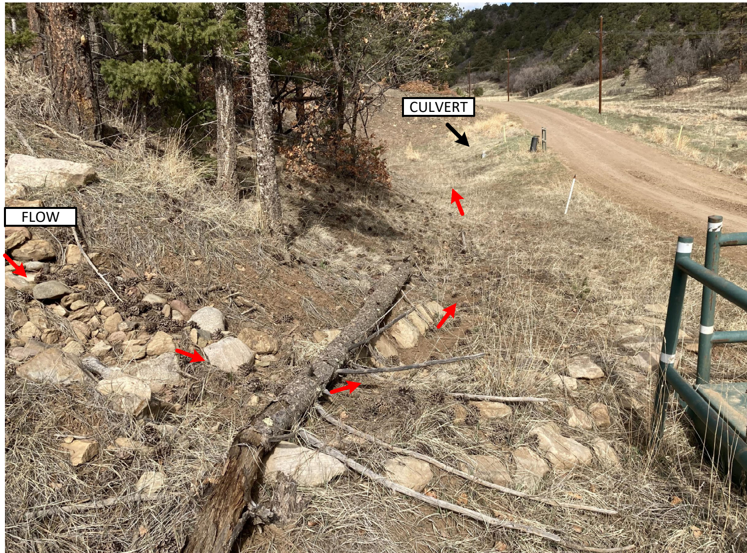
PHOTO 3: THE ARMORED CALL OUT DIRECTS RUN OFF FROM THE WELL PAD ACCESS ROAD TO A GRASSY SWELL WHICH WILL ALLOW SEDIMENT TIME TO DROP OUT. AFTER PONDING, RUN OFF WILL THEN ENTER A GALVANIZED CULVERT THAT CROSSES THE MAIN LEASE ROAD IN ALAMOSITO CANYON.
