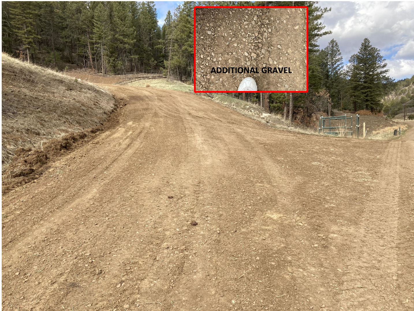
PHOTO 1: THE ROAD SURFACE WAS CROWNED TO CREATE SHEET FLOW AND ELIMINATE THE TIRE RUTS. ADDITIONAL GRAVEL WAS ADDED TO THE ROADWAY SURFACE FOR STABILIZATION.
