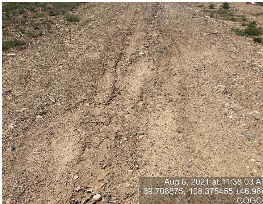
Access road erosion/lack of stabilization/compaction
