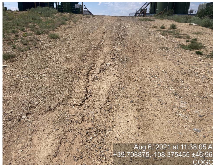
Access road erosion/lack of stabilization/compaction
