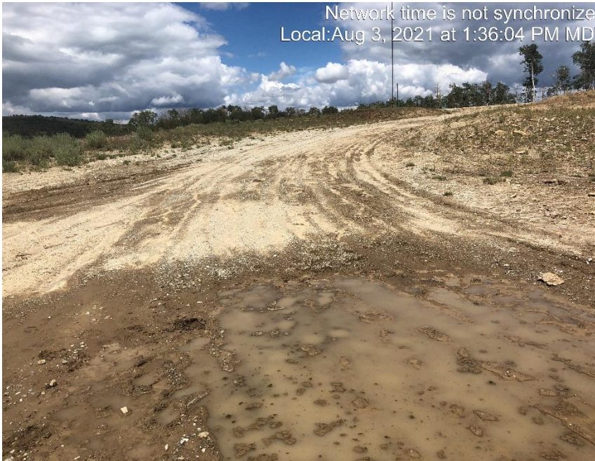
Photo #4672 No form of tracking BMP located at entrance to location.
