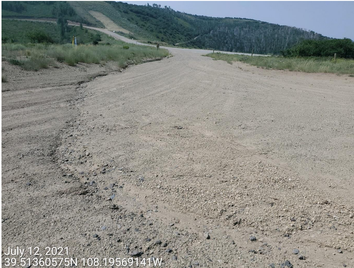
Photo 12: Photo taken from the access road, south of the Location. Photo shows stormwater erosion degradation on access road due to runoff from the Location.
