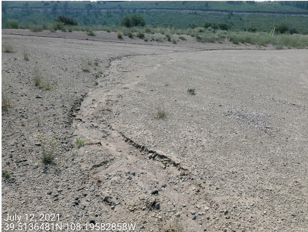
Photo 11: Photo taken from the Location entrance (south end of the Location), facing southeast. Photo shows stormwater runoff from the Location has resulting in erosion degradation on the access road, and off-site sediment transport.
