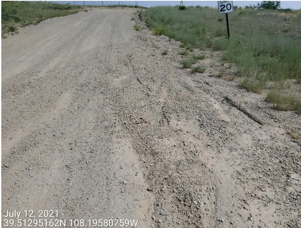
Photo 14: Photo taken from the access road. Photo shows sediment deposition resulting from stormwater runoff from the Location and erosion degradation.
