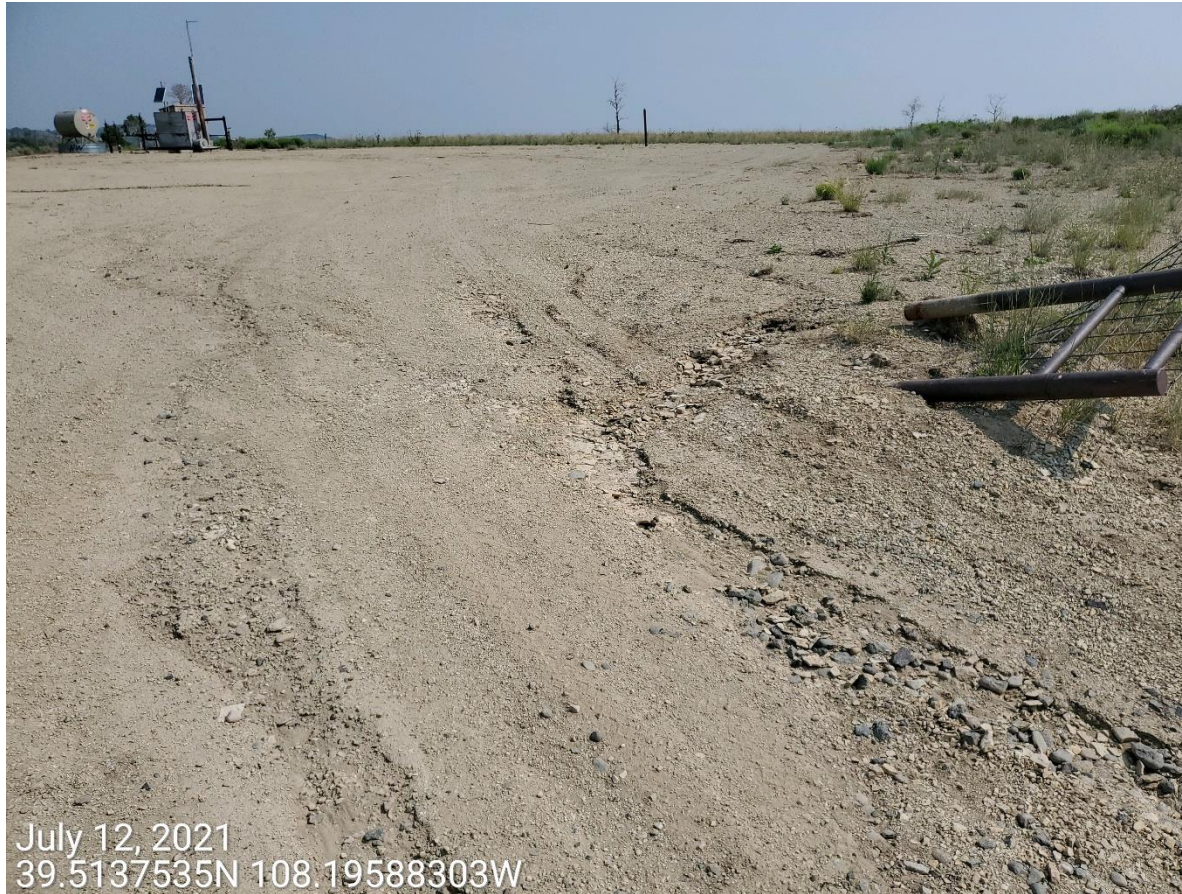
Photo 8: Photo taken from the Location entrance (south end of the Location), facing north. Photo shows erosion degradation due to stormwater runoff from the pad; stormwater runoff has resulted in erosion degradation and offsite sediment discharge at Location entrance and access road.
