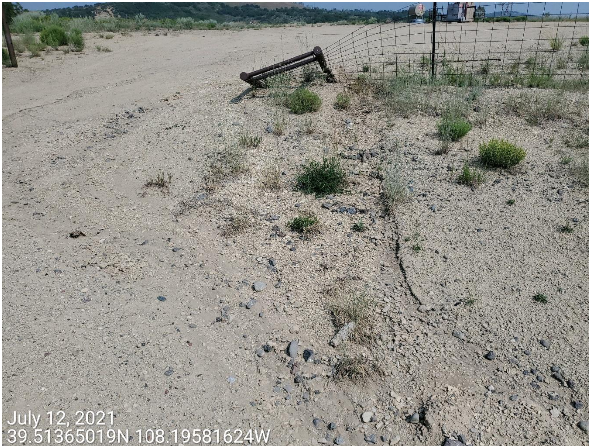
Photo 10: Photo taken from the Location entrance (south end of the Location), facing north. Photo shows erosion degradation due to stormwater runoff from the pad
