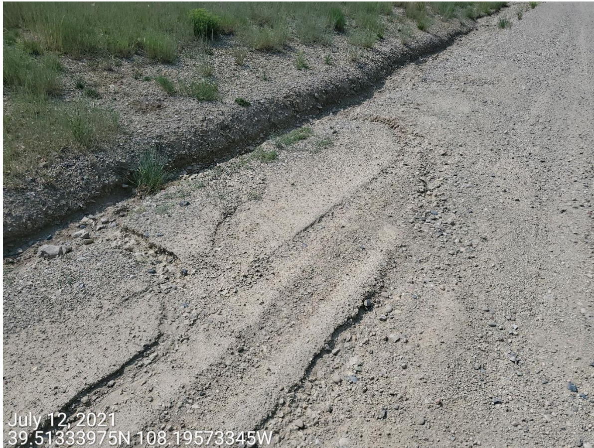
Photo 13: Stormwater erosion on access road.
