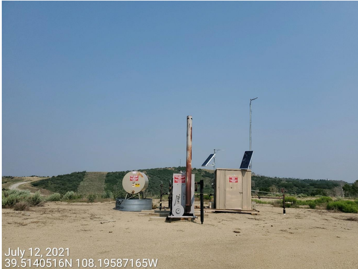
Photo 4: Photo facing west. Photo shows metershed, separator equipment and methanol tank. Photo also shows bird protector equipment appears to be missing from top of the separator.
