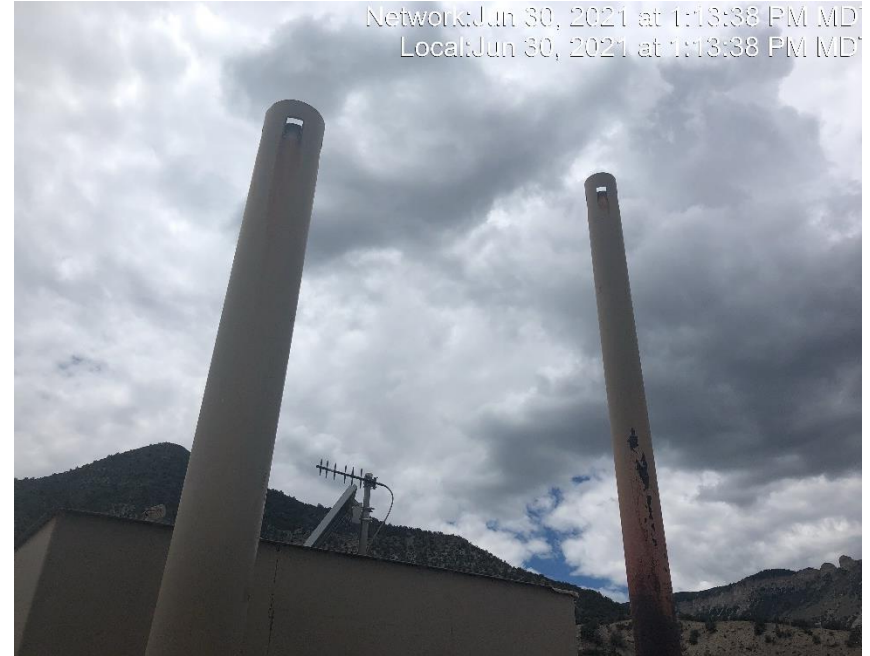
Photo #4244 Bird protectors missing on separator.
