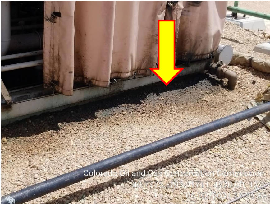
Photo 11 – Stained Soil at Compressor
