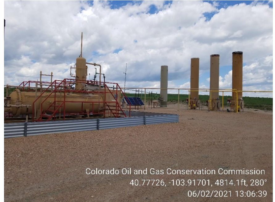
Photo 4 – Separators and ECDs
