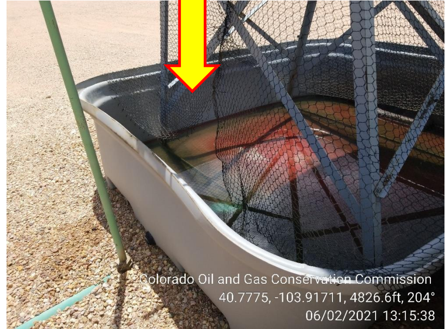
Photo 10 – Day Tank Netting inadequate
