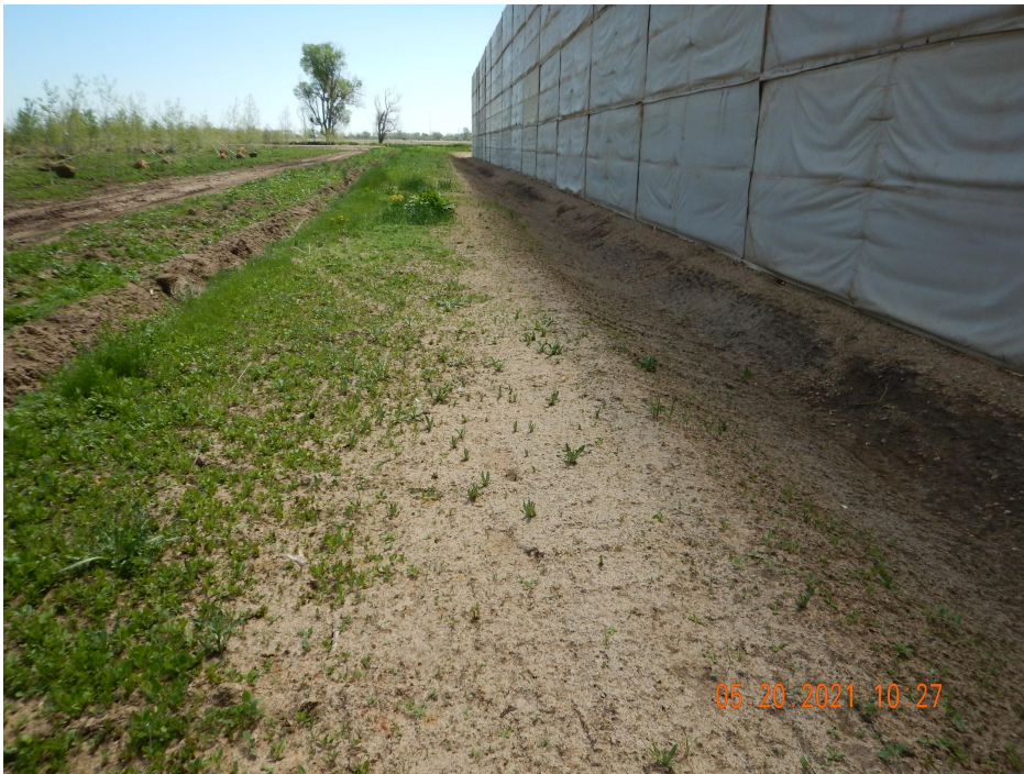
Photo 1. Photo taken from the northern location, facing East. Photo illustrates a cut slope that has been seeded and hydromulched.
