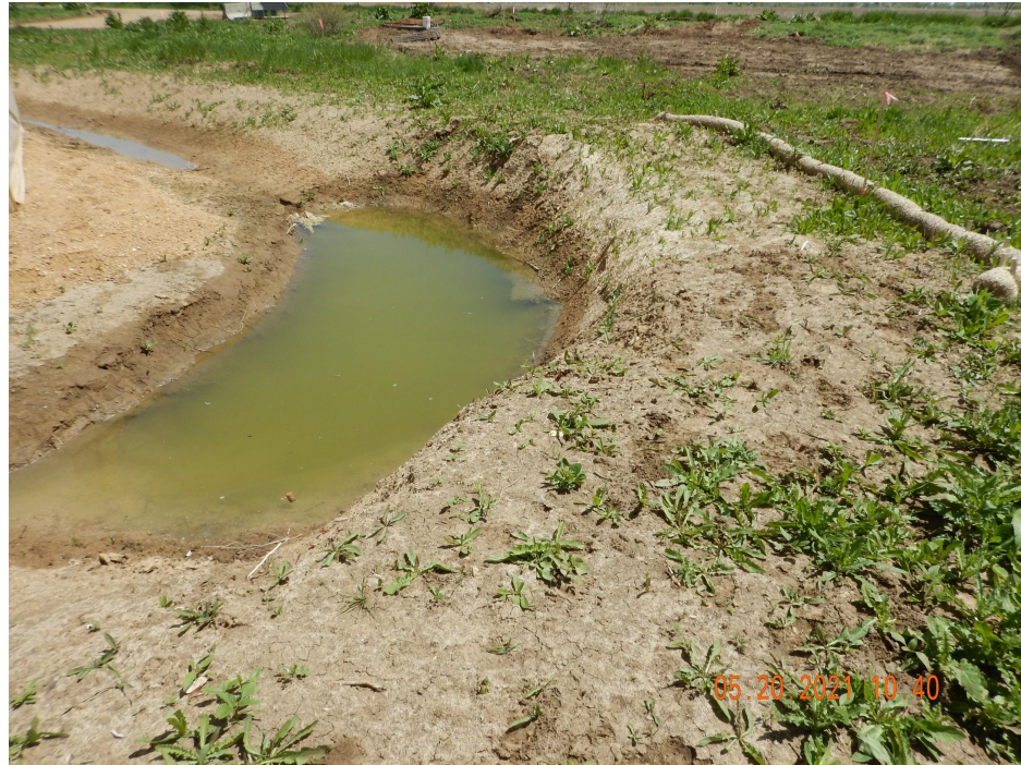
Photo 6. Photo taken from the southeastern location, facing Northeast. Photo illustrates a sediment trap with a temporarily stabilized outlet.
