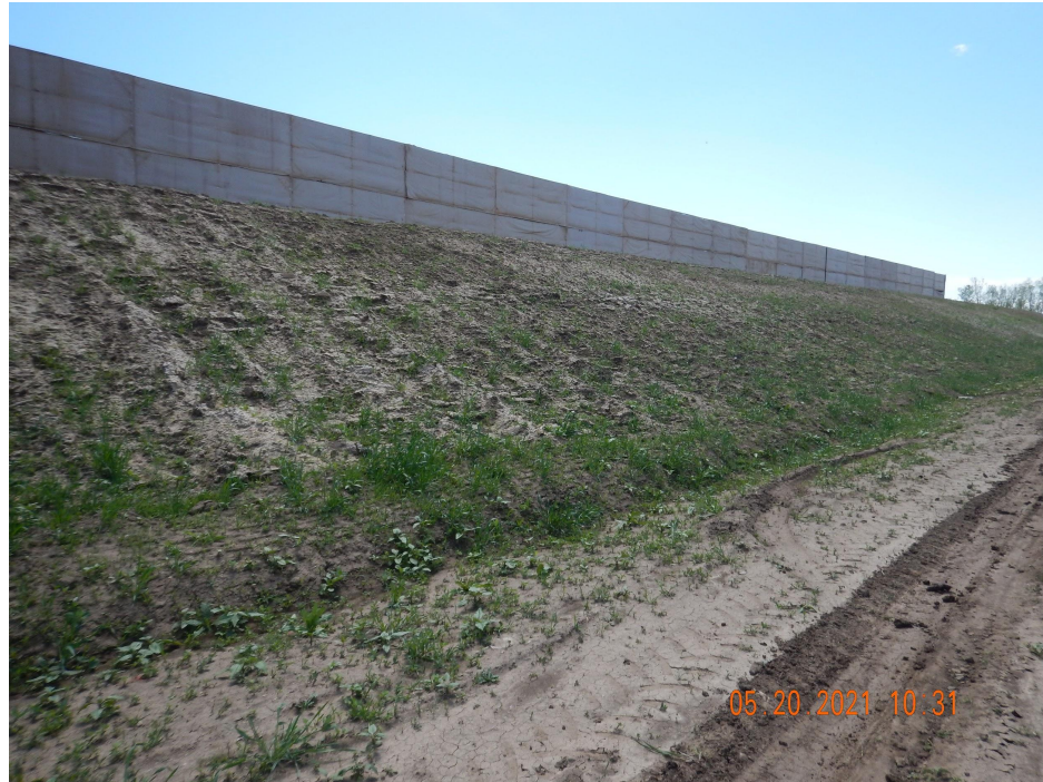
Photo 4. Photo taken from the western location, facing Southeast. Photo illustrates the topsoil stockpile has been tracked, seeded and hydromulched. Germination of desirable plant species were observed throughout most of the stockpile. There was a bare area along the southern stockpile.
