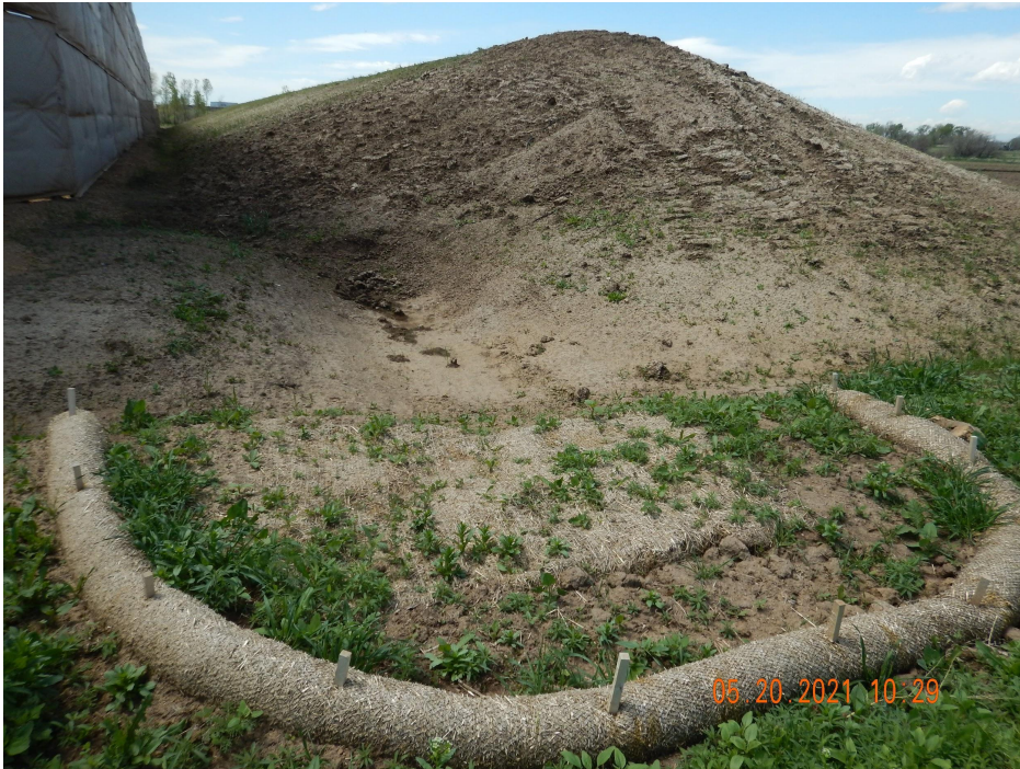
Photo 3. Photo taken from the northwestern location, facing South. Photo illustrates a stormwater BMP and the topsoil stockpile.
