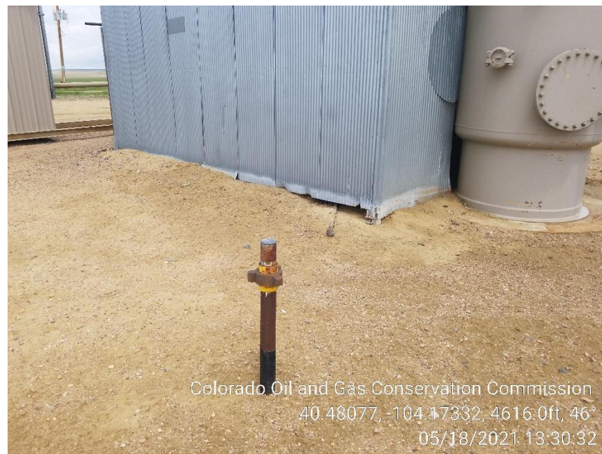
Photo 6 – Unmarked Riser at Heater
