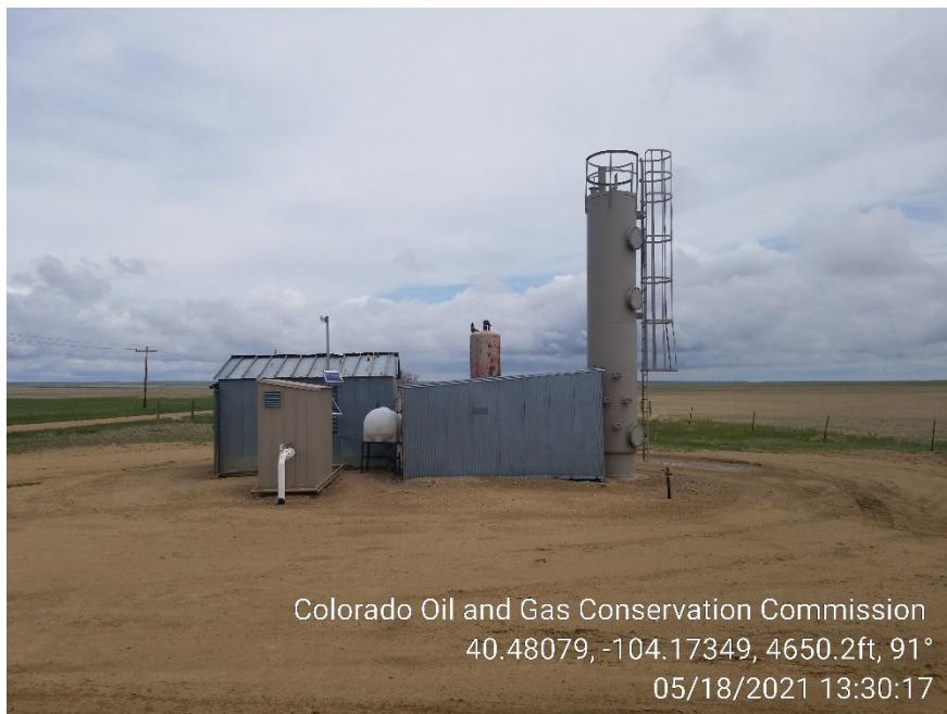
Photo 3 – Heater Treater
