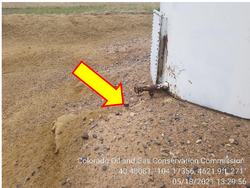
Photo 9 – Unmarked Risers at the back of the West Tank
