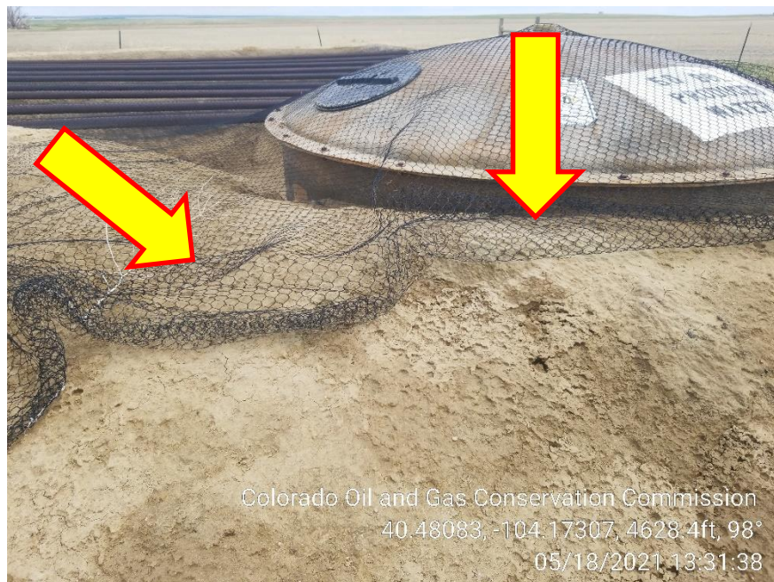
Photo 13 – Netting at Pit NOT Secure. Wildlife Hazard
