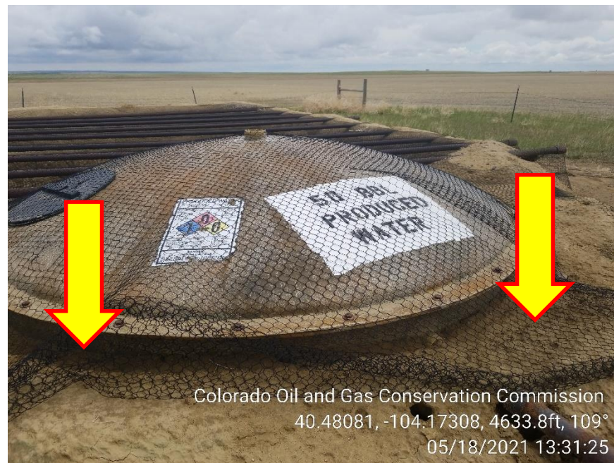
Photo 12 – Netting at Pit NOT Secure. Wildlife Hazard
