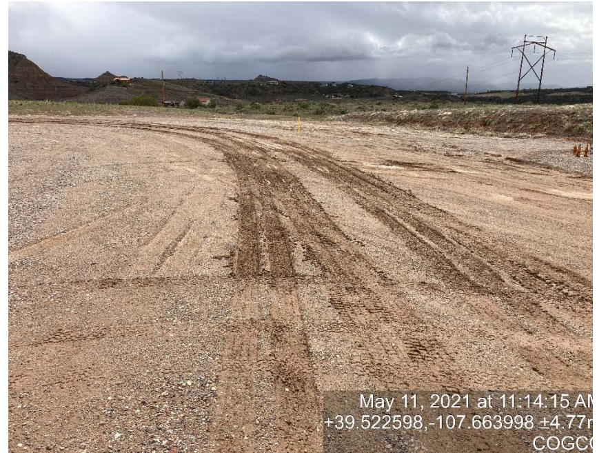
Lack of stabilization/compaction
