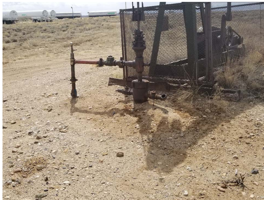
Photo 3. No bradenhead access apparent.
