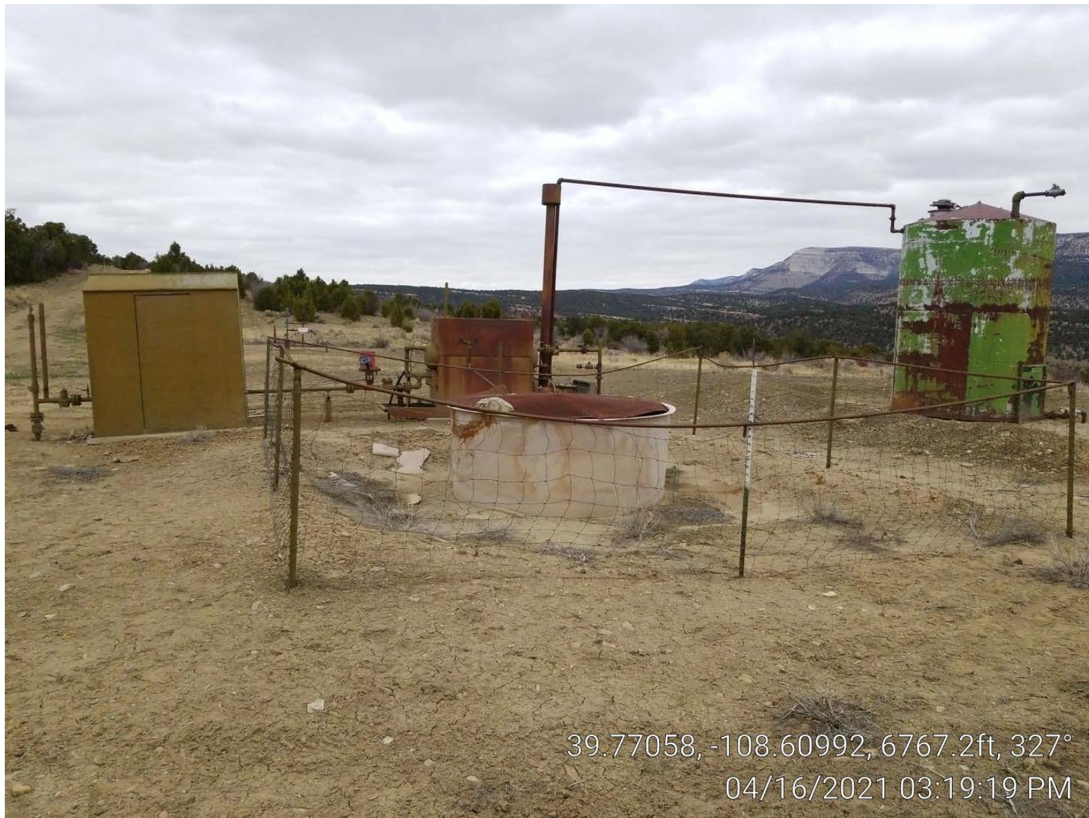
Photo 3. Meter building, separator, tanks.
