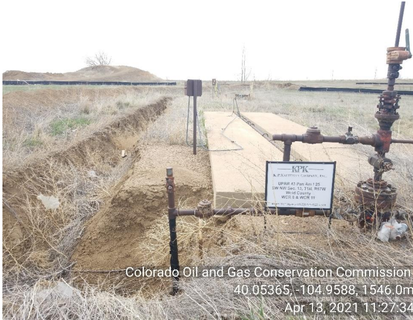
Photo 3 Site Remediation: Pipeline open excavation has been open since 4-4-18.
