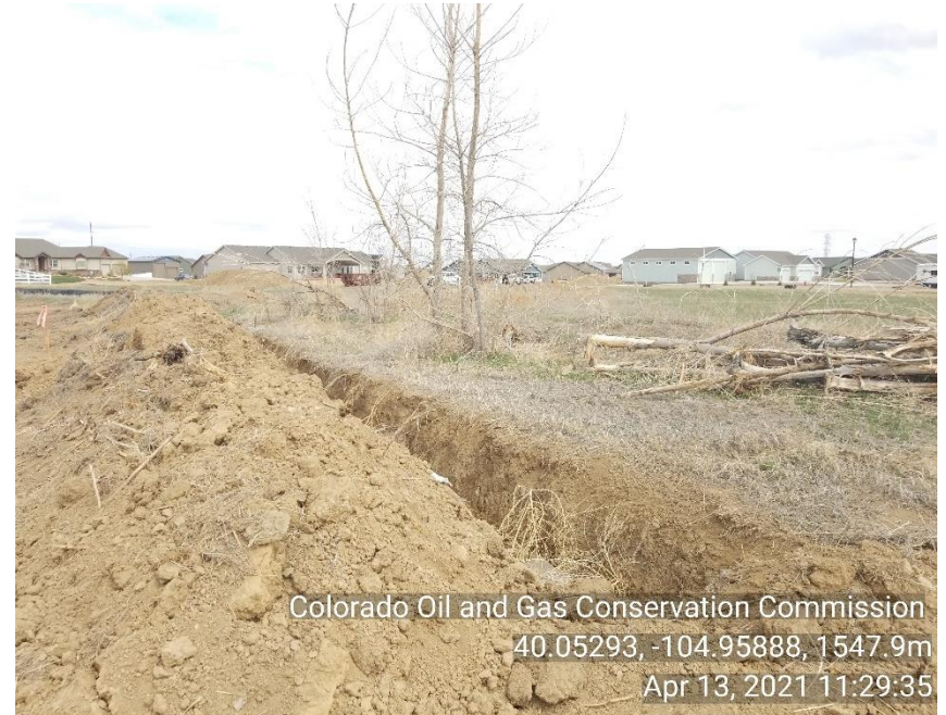
Photo 6 open excavation no BMP's.
