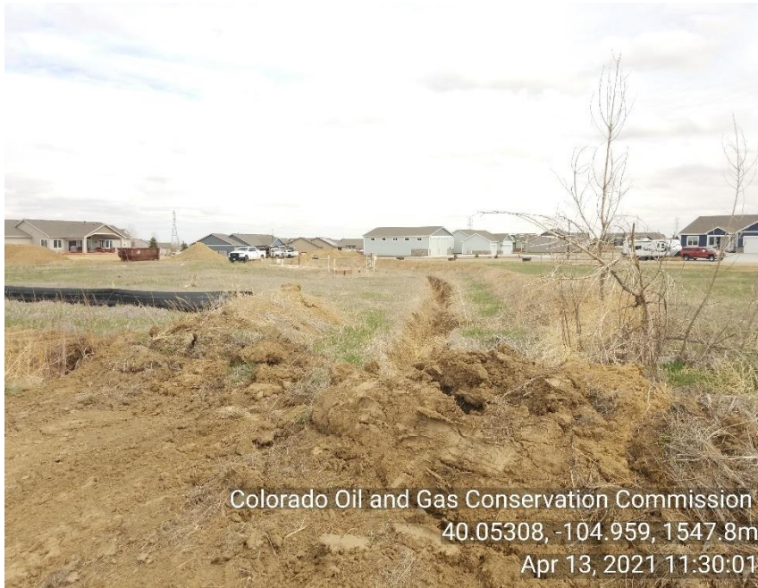
Photo 7 open excavation facing North. No fencing and or BMP's.
