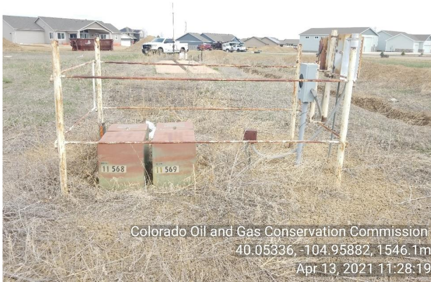
Photo 5 Unused equipment: electric panel, Meter has been removed.
