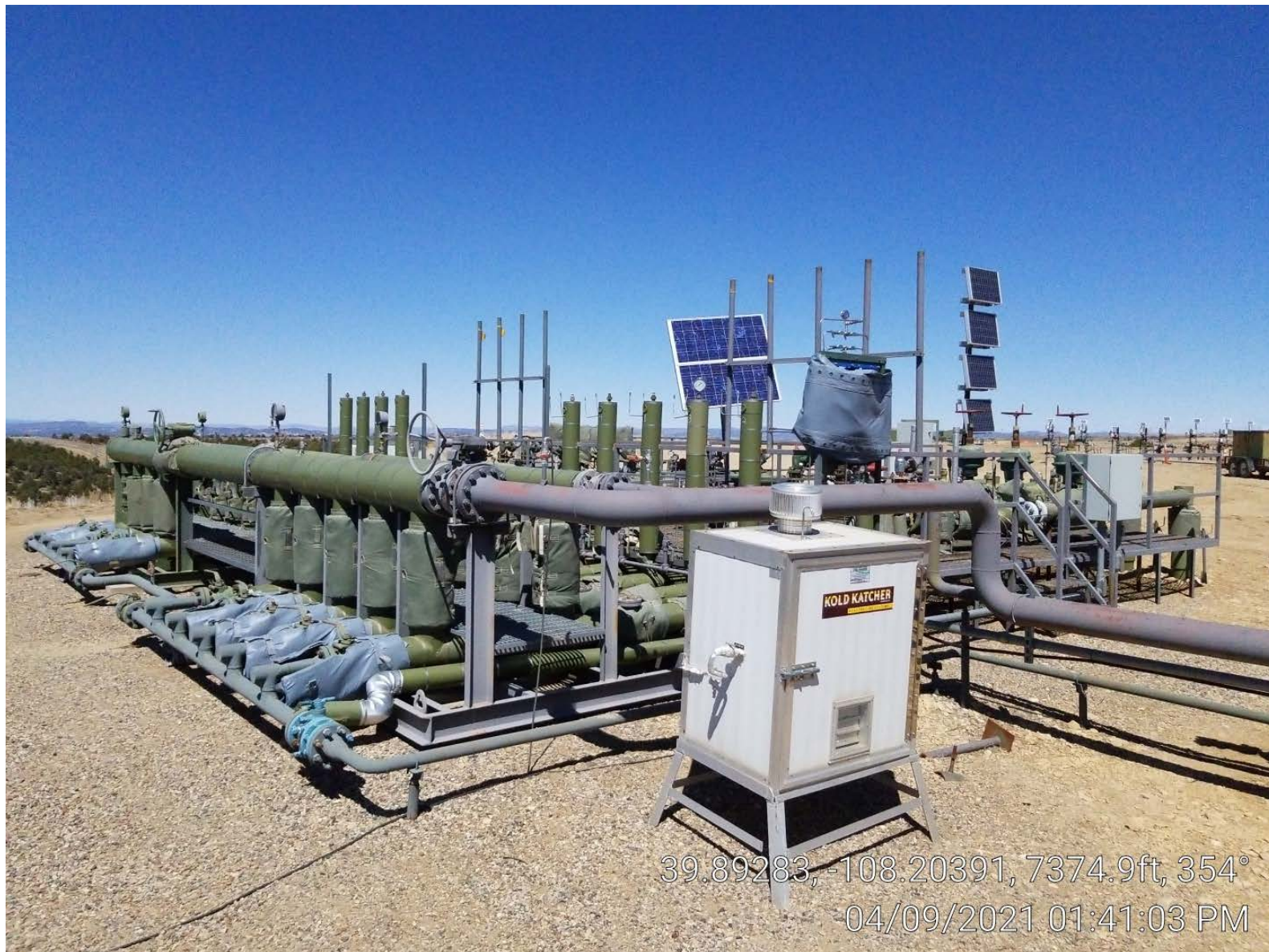
Photo 4. Well manifold.
