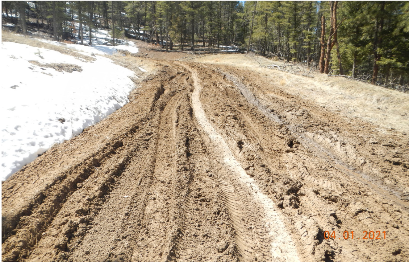
Photo 1. Facing toward the access road. The access road is rutted and not stabilized and maintained.
