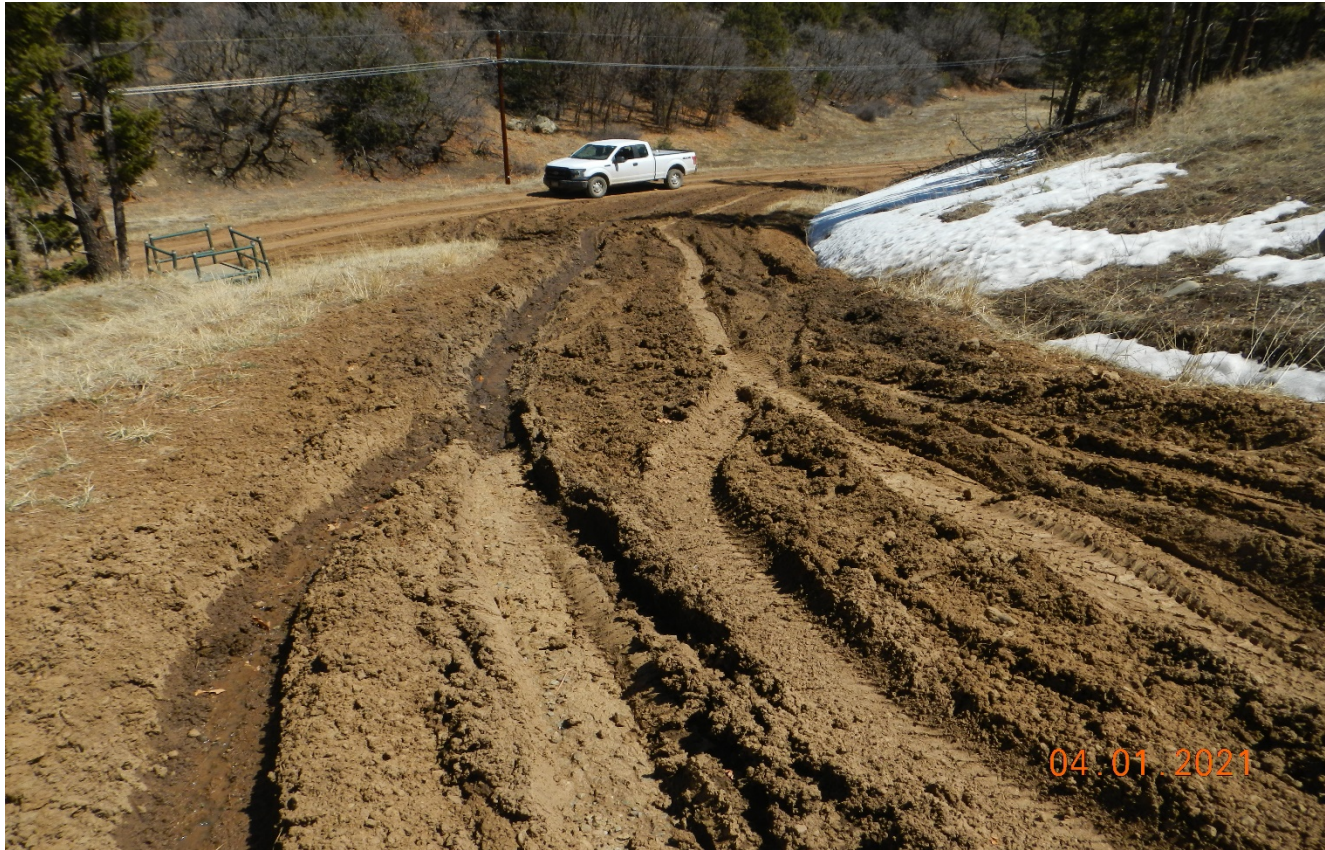
Photo 2. Facing back down toward the access road. The access road is rutted and not stabilized and maintained.
