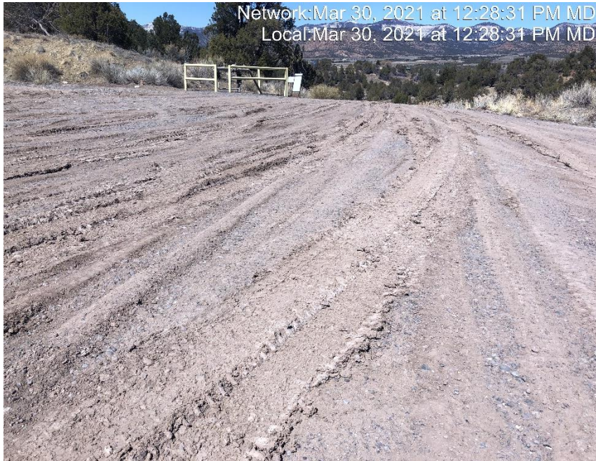
Photo #3333 No form of tracking control at entrance to location
