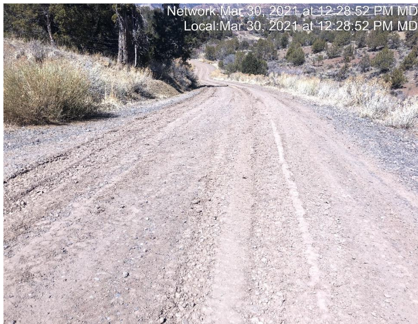
Photo #3334 No form of tracking control at entrance to location.
