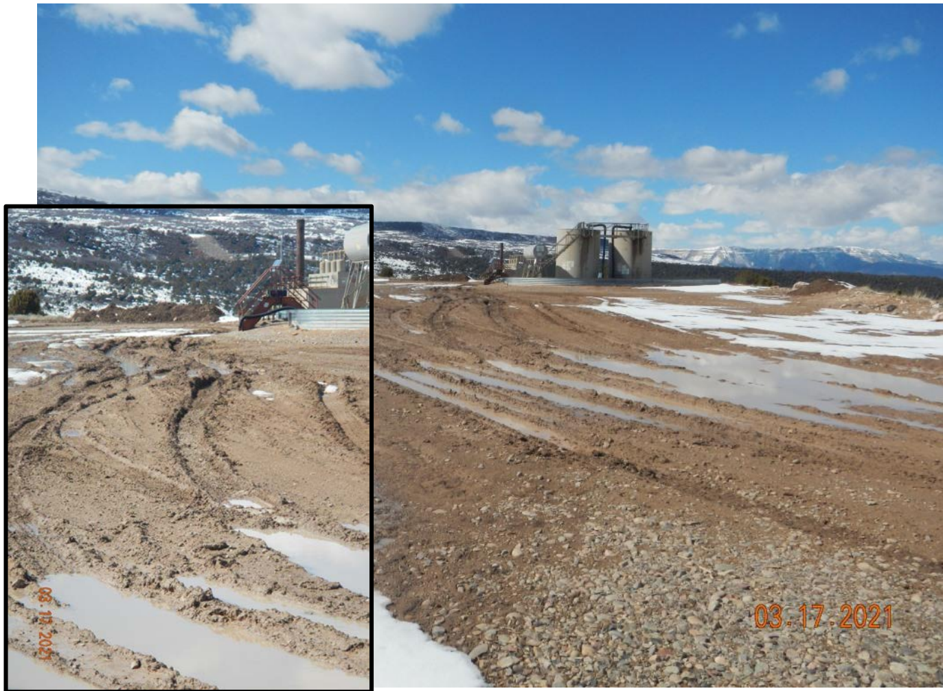
Photo#1: Overview of Location. Insert, rutting, unstable working surface.
