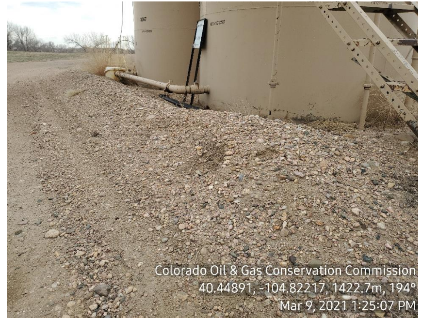
Photo 12: Inadequate berm
