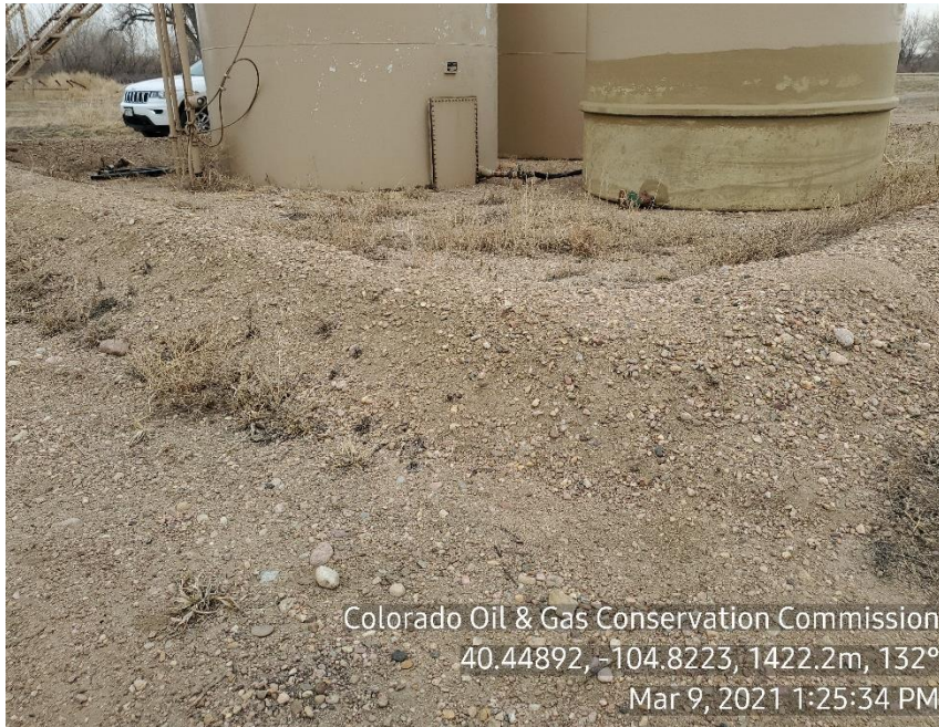
Photo 13: Inadequate berm
