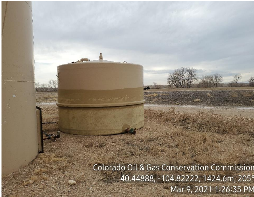
Photo 11: No contents/capacity/NFPA placard on tank
