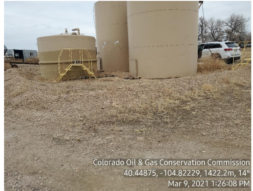
Photo 14: Inadequate berm
