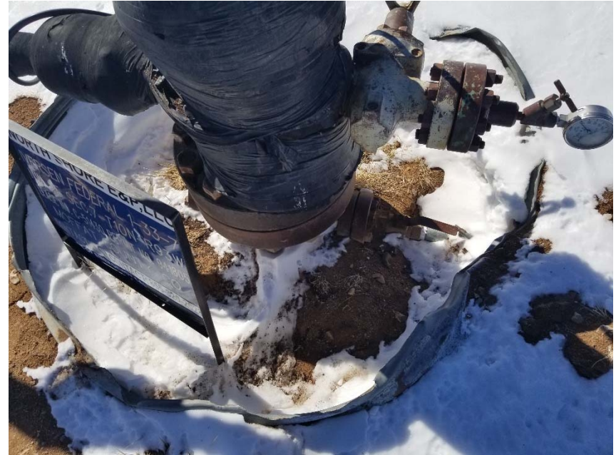
Photo 2. Bradenhead access installed.
