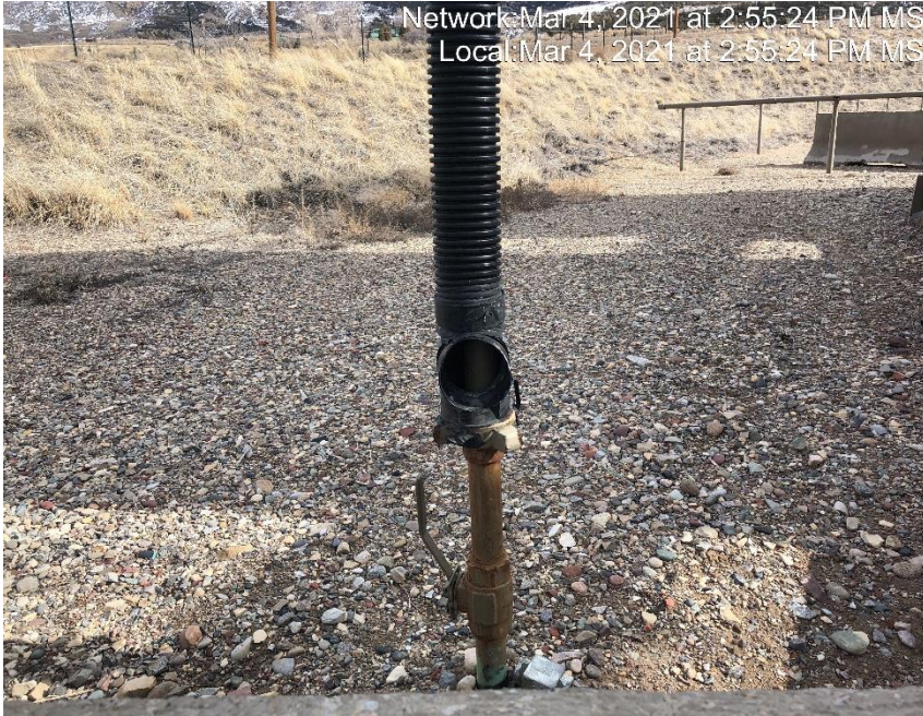
Photo #3061 Flow line heating insulation open ended and not capped.
