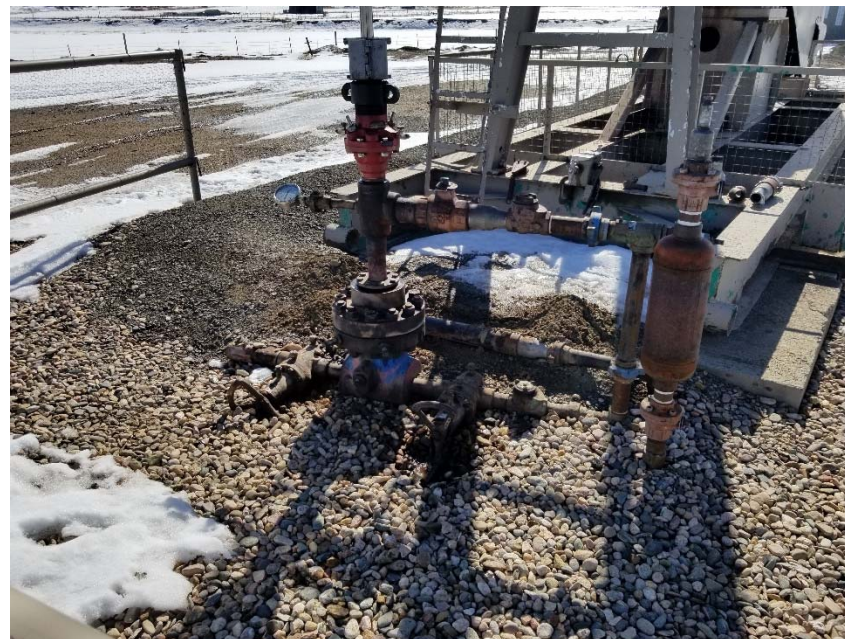
Photo 3. No bradenhead access apparent.
