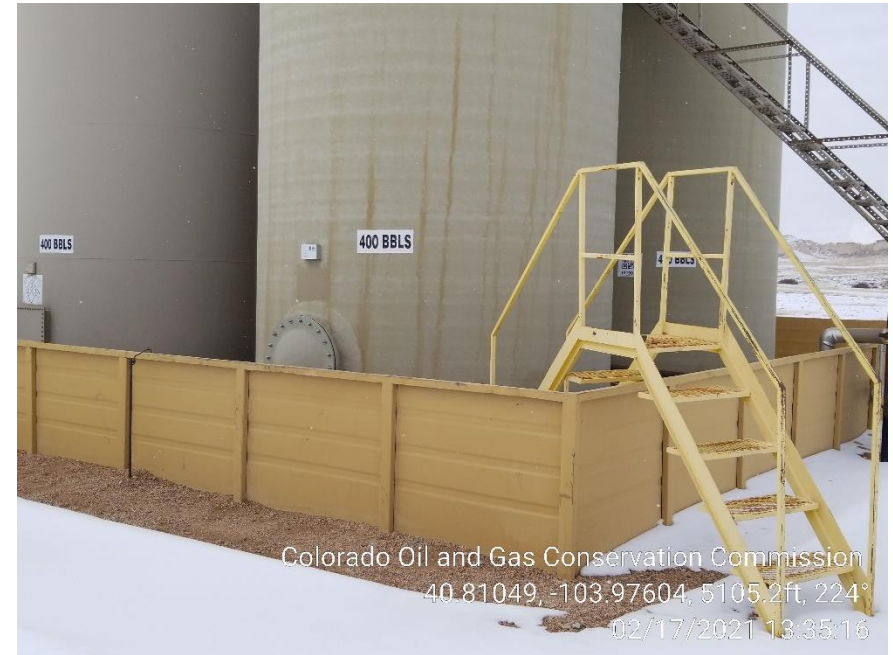
Photo 4 – SE Water Tank missing NFPA label
