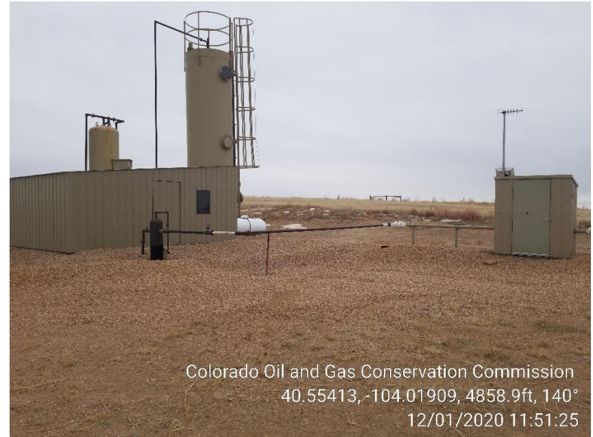
Photo 2 – Heater Treater
