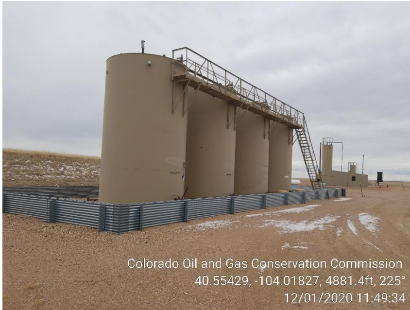
Photo 1 – Tank Battery
