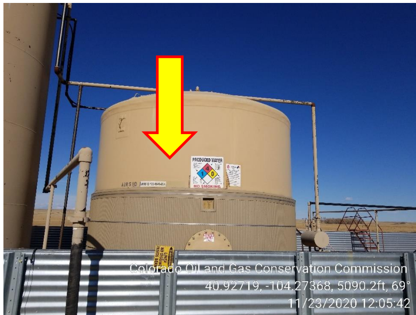
Photo 7 – Produced Water Tank Missing Capacity
