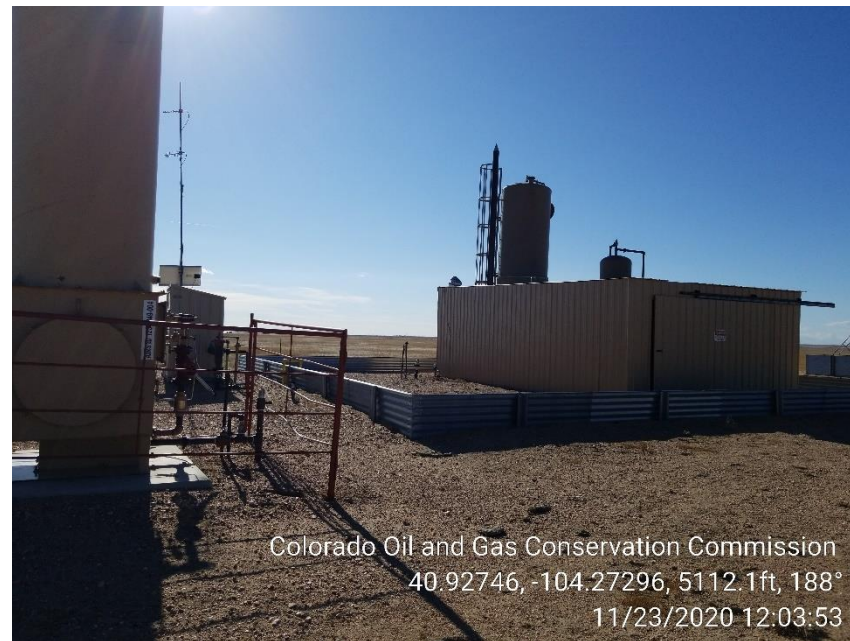
Photo 4 – Heater Treater, ECD
