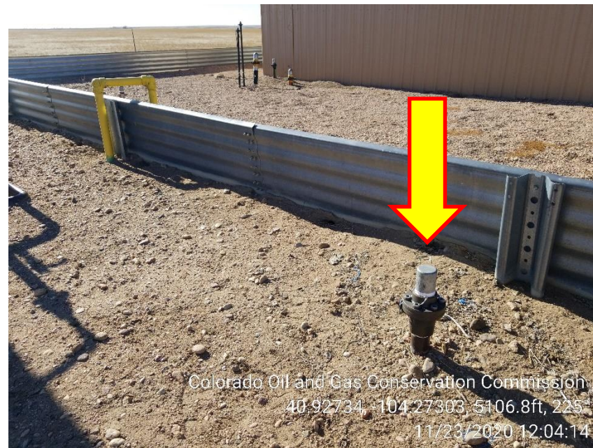
Photo 6 – Unmarked 2" Riser at Gas Meter
