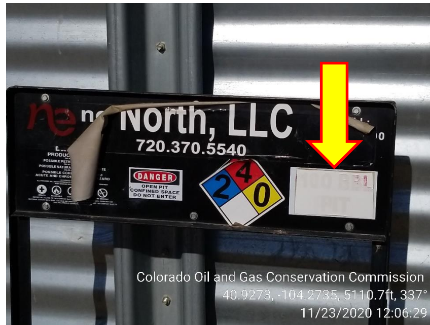
Photo 8 – Produced Water Tank Missing Capacity
